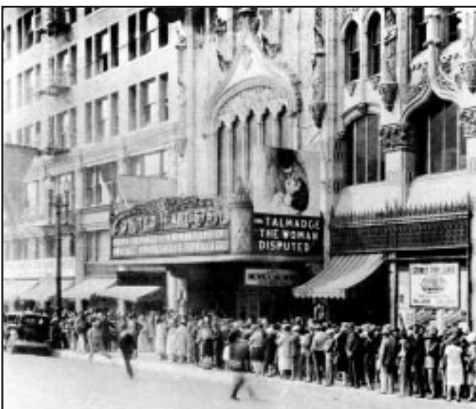
United Artists 933 Broadway Built 1927 Original Seating: ? seats Current Seating: 1,700 seats Current Use: Church
