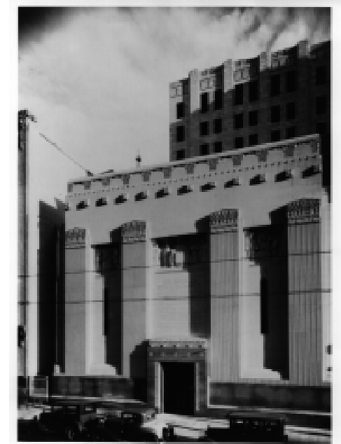
Los Angeles Stock Exchange Security Pacific National Bank Photo Collection Los Angeles Public Library
