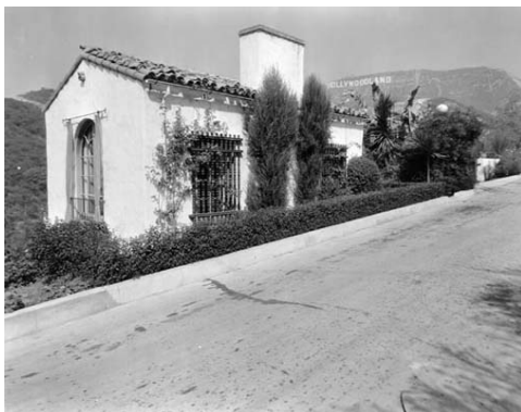
An original house after construction
