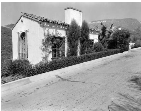
An original house after construction
