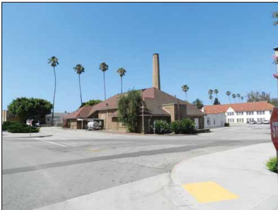
Photograph 22. Looking toward support facilities area showing Boiler House, Vector Control, and Barber/Beauty Shop; facing southwest, June 23, 2015. Notice the minimal vegetation and expanse of asphalt paved road, parking space, and loading/unloading area.
