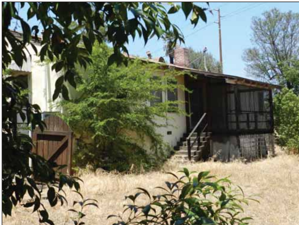
Photograph 5: Rear (south side) of Residence 17; facing northeast, June 23, 2015.
