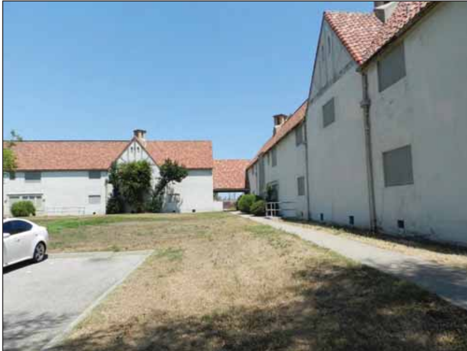
Photograph 2: Detail view showing breezeway; facing east, June 23, 2015.
