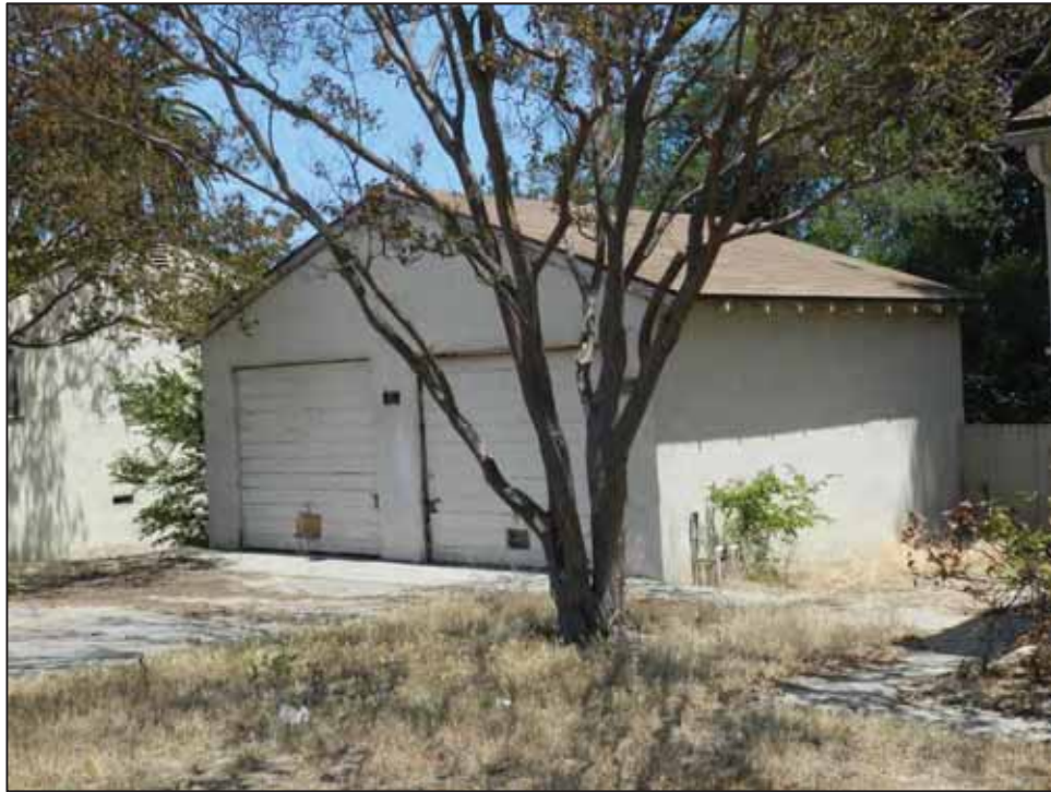
Photograph 10: North and west sides of Garage 16/17; facing northeast, June 23, 2015.
