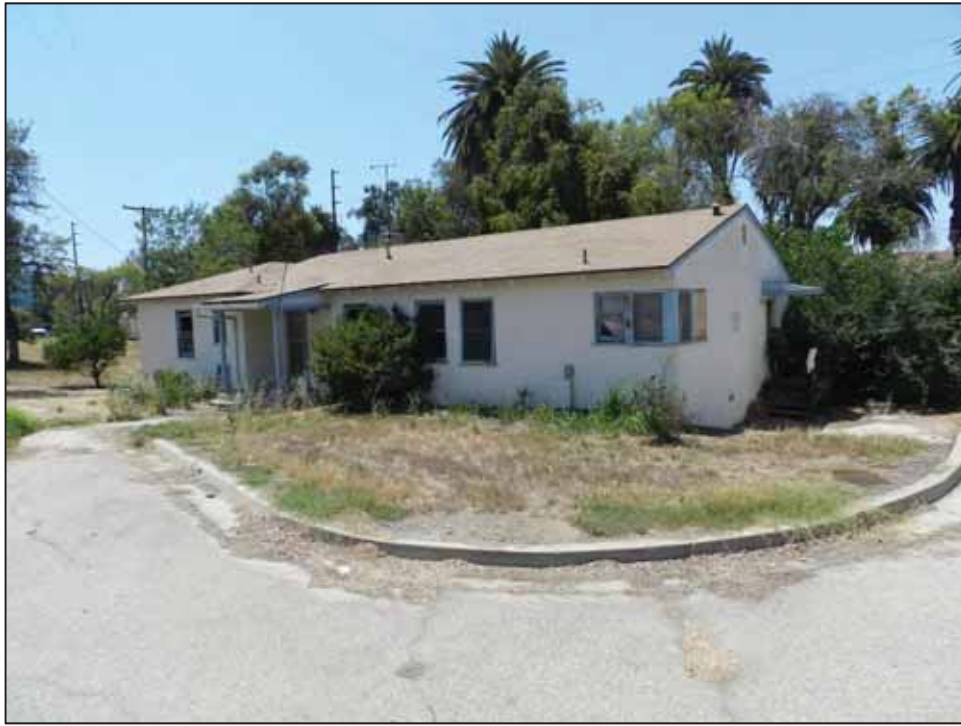
Photograph 8: Residence 19; facing northwest, June 23, 2015.
