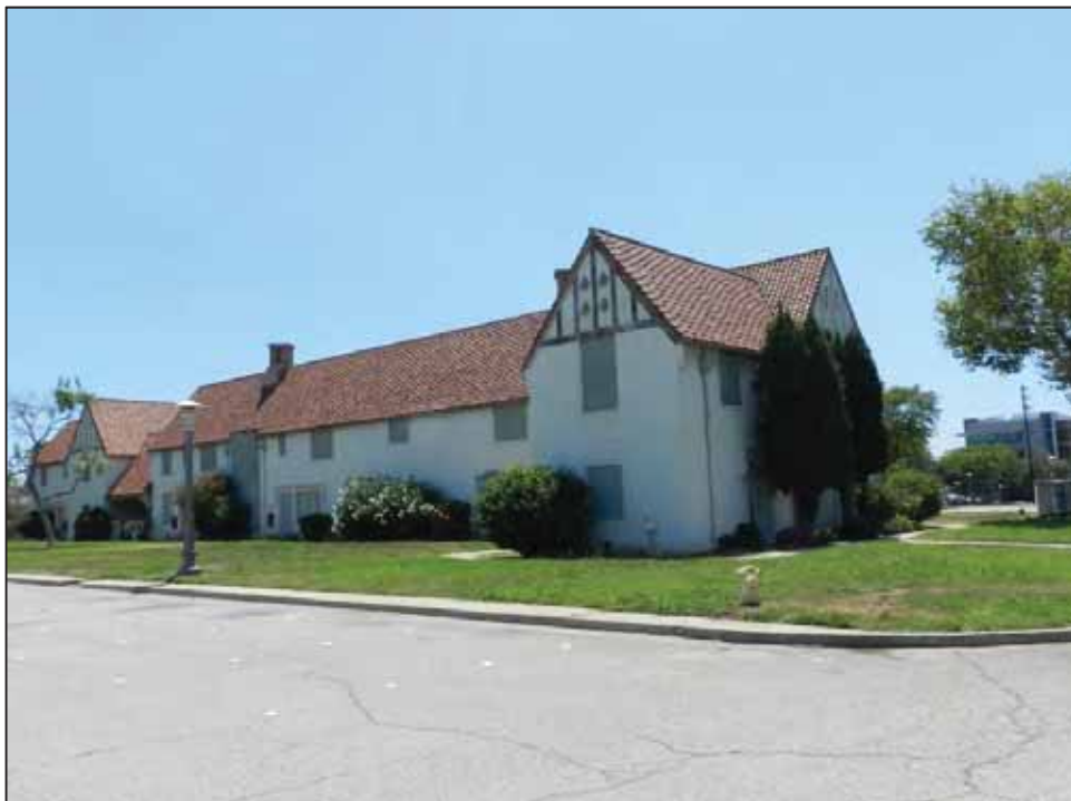
Photograph 3: North and east sides of Employee Building 3; facing southwest, June 23, 2015.
