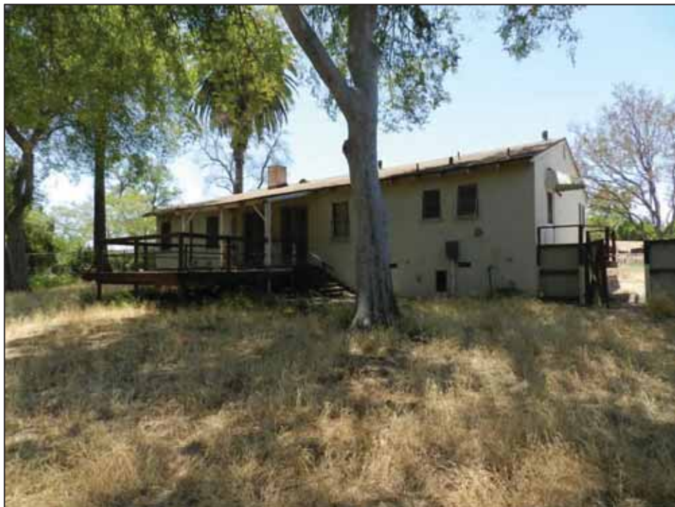
Photograph 3: Rear (south side) of Residence 16; facing northwest, June 23, 2015.
