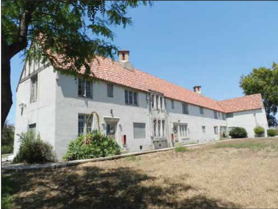
Photograph 4: West and south sides of Employee Building 4; facing northeast, June 23, 2015.
