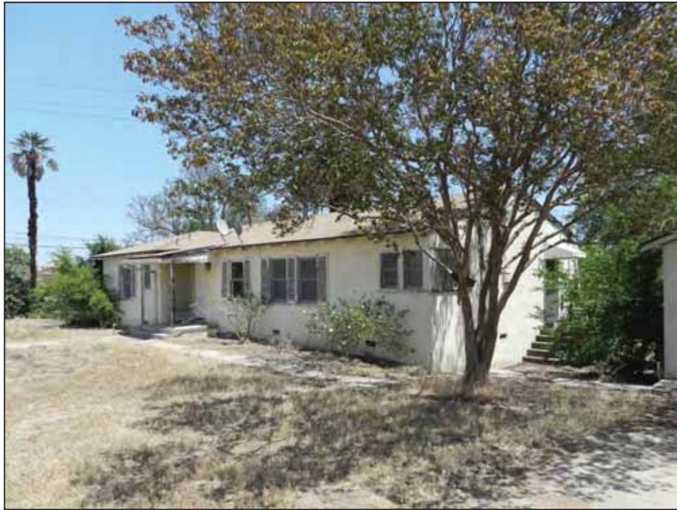
Photograph 4: North and west sides of Residence 17; facing northeast, June 23, 2015.
