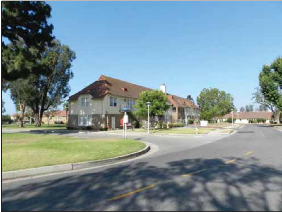
Photograph 3. Looking toward Birch Grove Homes from North Circle Drive near Res. 12; facing southwest, June 23, 2015.
