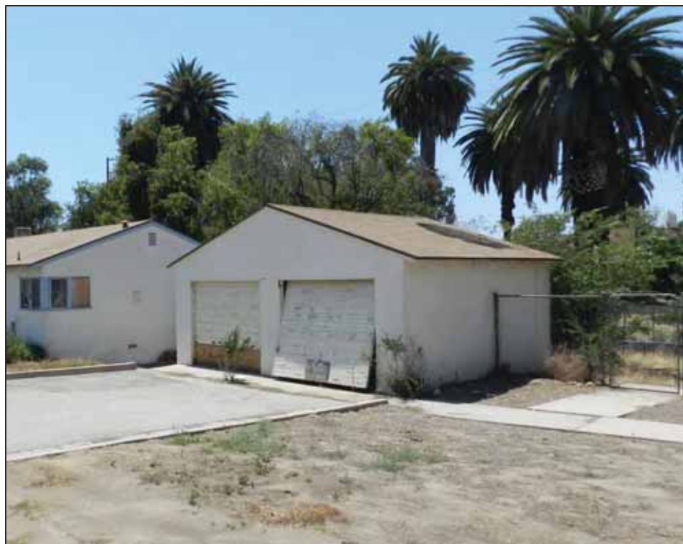
Photograph 11: South and east sides of Garage 18/19; facing northwest, June 23, 2015.
