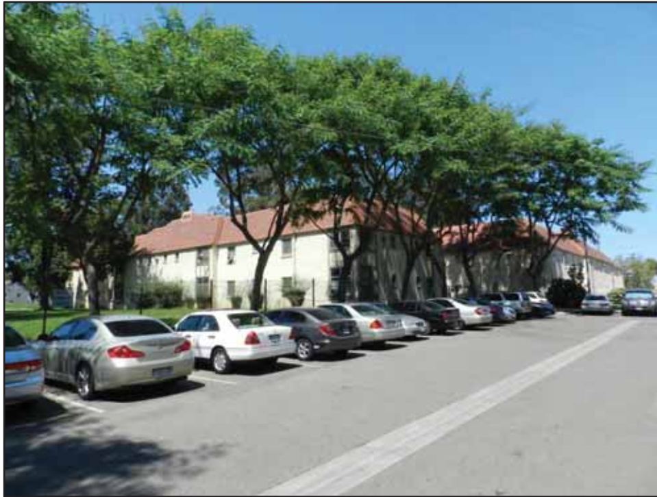
Photograph 21. Employee Buildings 1 and 2; facing northeast, June 23, 2015.
