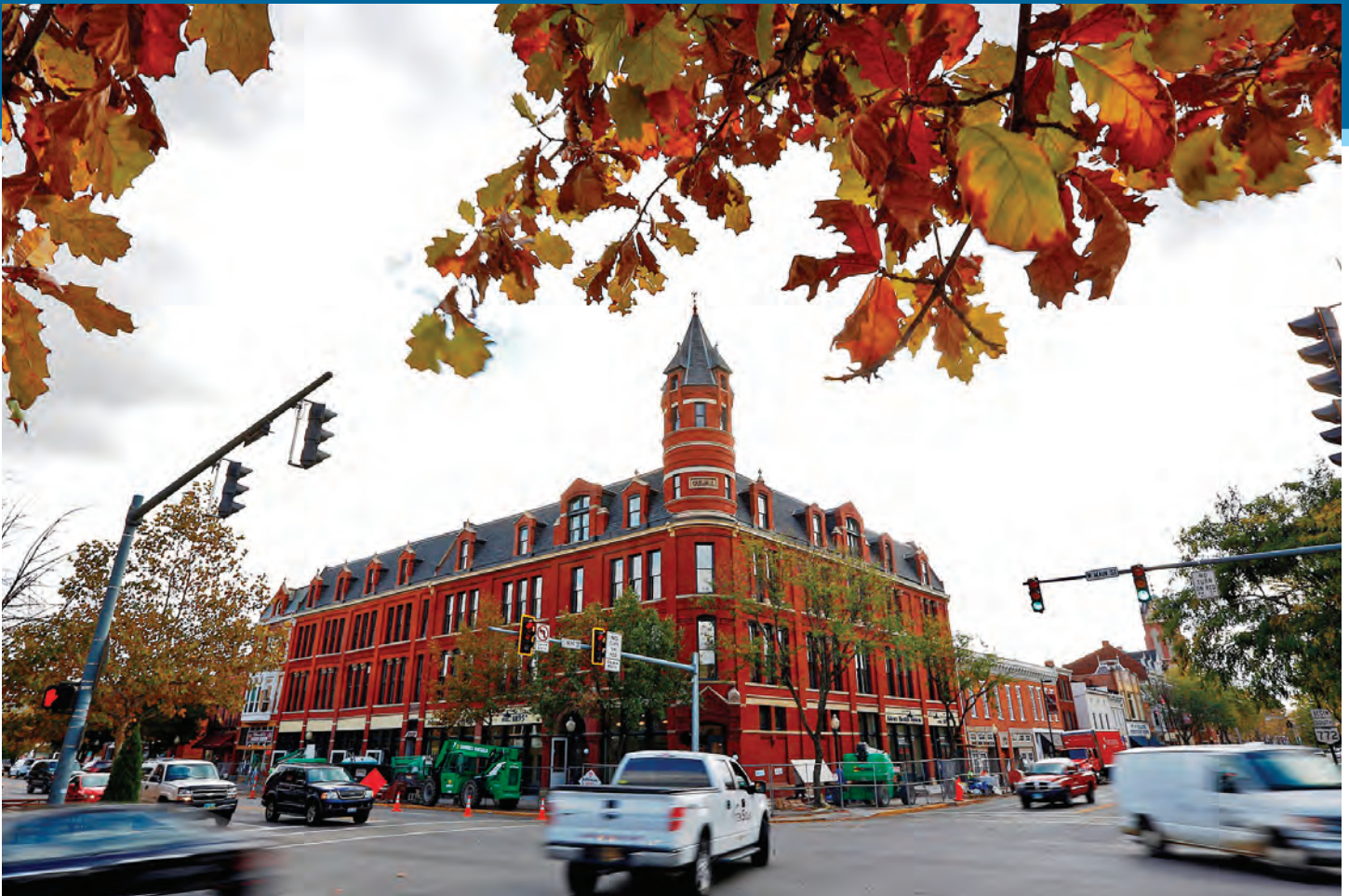
Nearly destroyed by fire and covering almost a city block, the 1895 Carlisle building in Chillicothe (pop. 21,700) now offers office space on the ground floor and 32 loft apartments for medical professionals in the upper floors.
