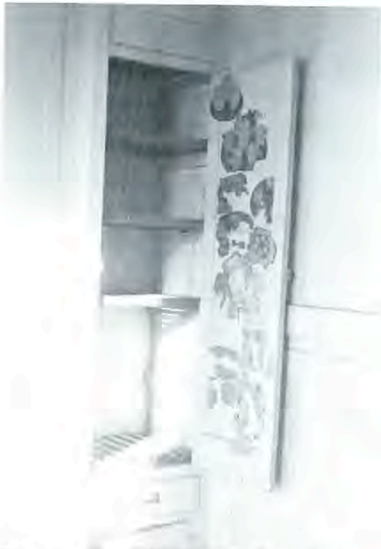
The kitchen cupboard is cooled by vented outside air.
