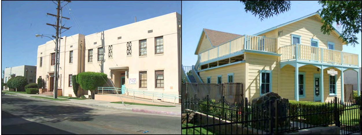
Figure 8. Previously recorded cultural resources within the planning area. Left: the Cedar Avenue Complex; right: the Western Hotel.
