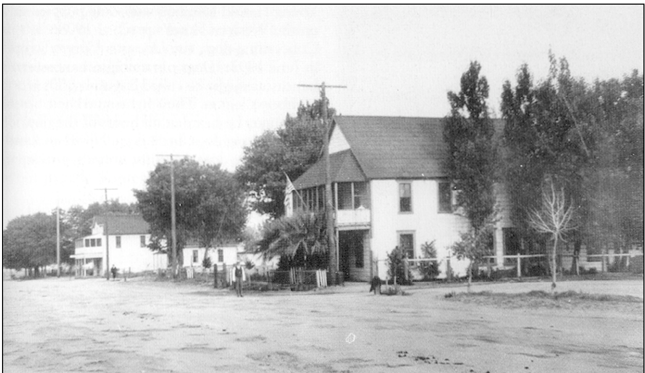
Figure 3. Lancaster Boulevard, ca. 1910 (view to the northwest from Antelope Avenue, now Sierra Highway). (Source: Gurba 2005:93)
