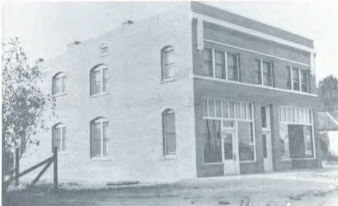
The 1923 Ledger-Gazette regarded the building “in every sense of the word a credit to the town and community.”
