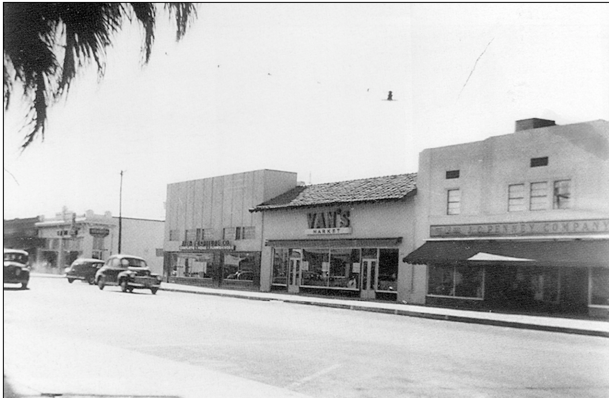
Figure 5. Lancaster Boulevard around Beech Avenue in the early 1950s (view to the southeast). (Source: Gurba 2005:60)
