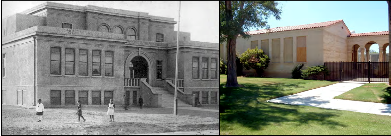
Figure 12. The former Lancaster Grammar School (left, view to the northwest; Gurba 2005:29), built in 1913, has been significantly altered and incorporated into a group of buildings housing the Lancaster School District offices today (right, view to the southwest).
