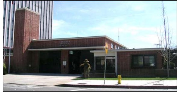
Fire Station, 3430 E. Foothill Blvd, 1952.
