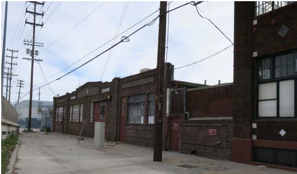
2415 S. Santa Fe Ave., east façade, view southwest (ARG, 2019).
