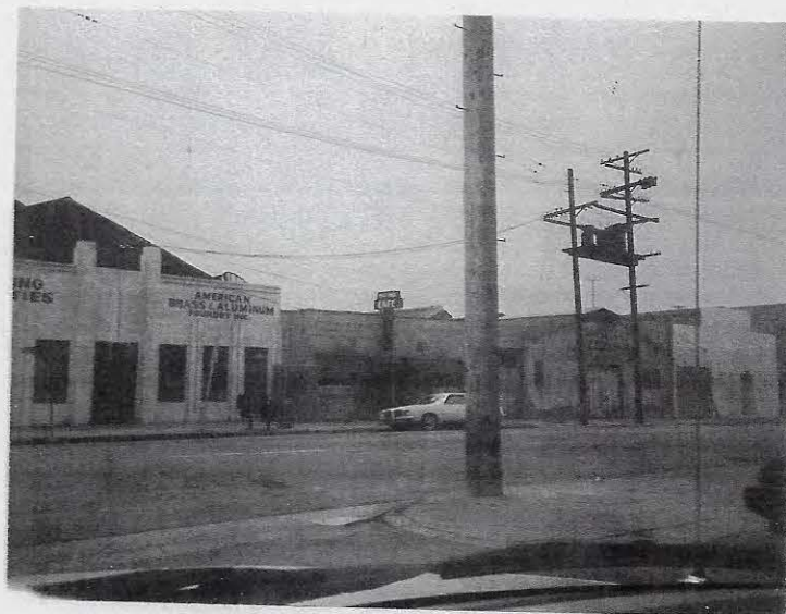
LOOKING SOUTHEAST, ACROSS SANTA FE AVE. TOWARD INDUSTRIAL BUILDINGS EAST OF THE SUBJECT PROPERTY
