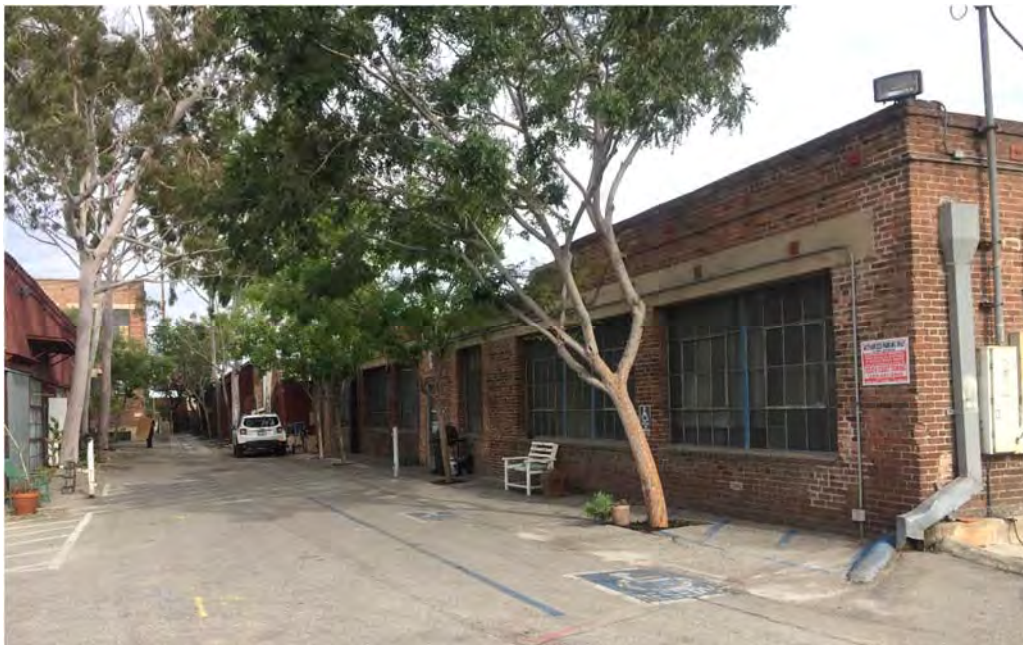
2421 S. Santa Fe Ave., north façade, view southeast (ARG, 2019).
