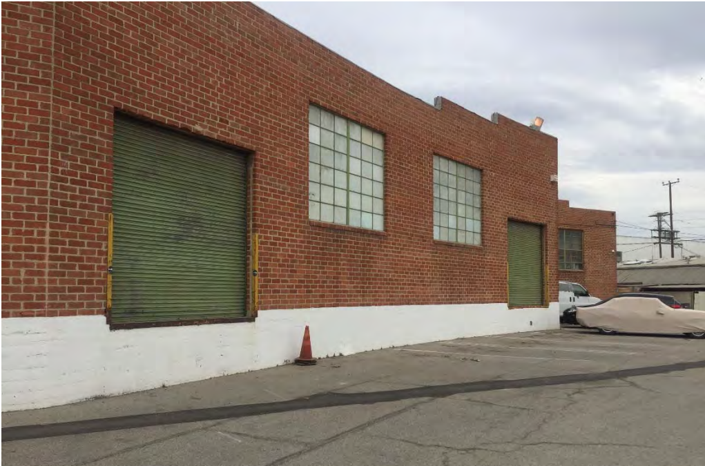
2345 S. Santa Fe Ave., south façade, view north (ARG, 2019).
