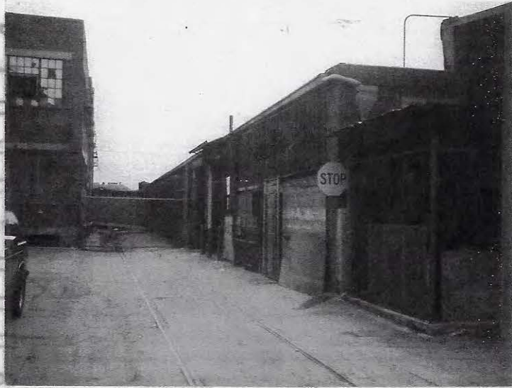
LOOKING EAST ALONG NORTH SIDE OF BUILDING AT 2421 SANTA FE AVE PROPOSED FOR FOUR UNITS (PHASE 2)
