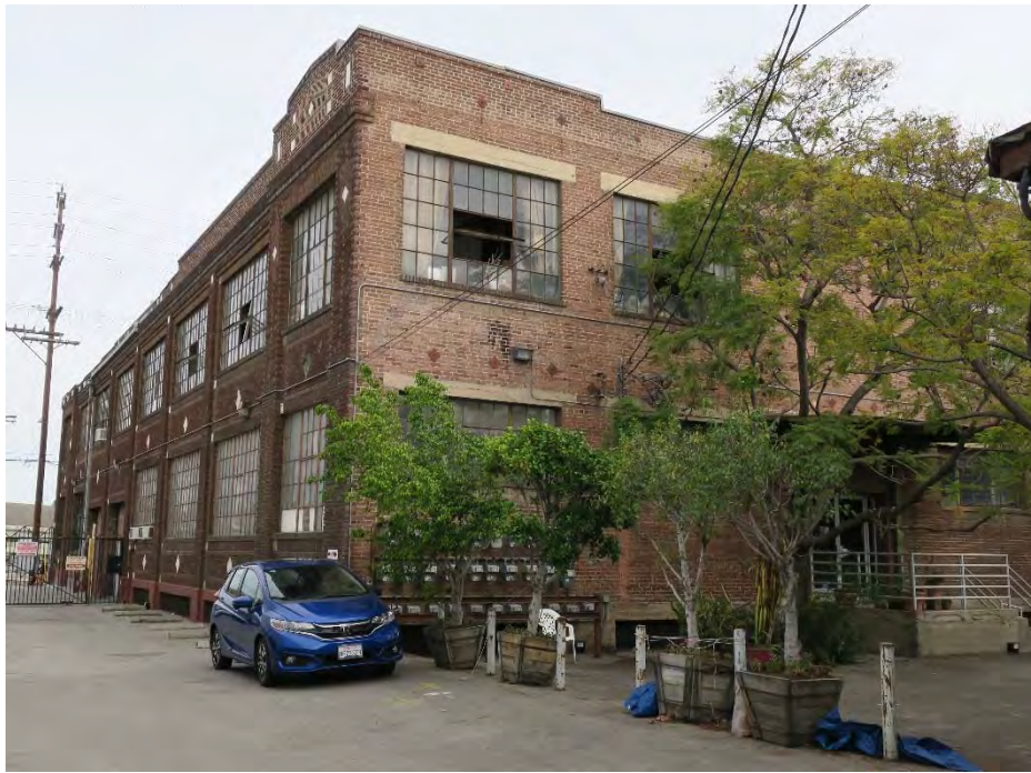
2401 S. Santa Fe Ave., north and west façades, view southeast (ARG, 2019).
