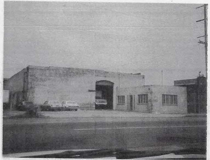
LOOKING NORTHWEST TOWARD INDUSTRIAL BUILDING ADJACENT TO, AND SOUTH OF, THE SUBJECT PROPERTY
