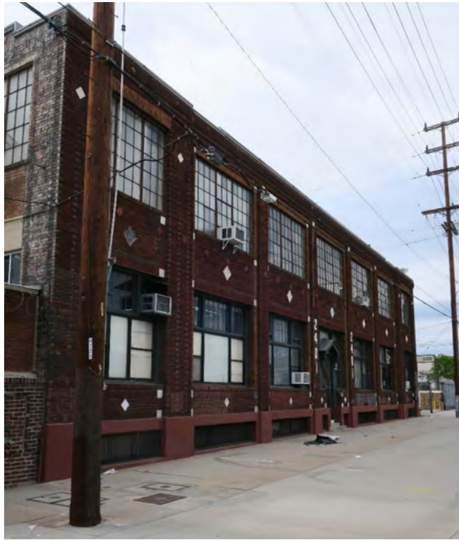
2401 S. Santa Fe Ave., east façade, view northwest (ARG, 2019).
