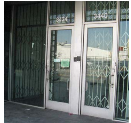
Interior grills that are more than 75% open are less visible during non-business hours and easier to screen from view during business hours.
