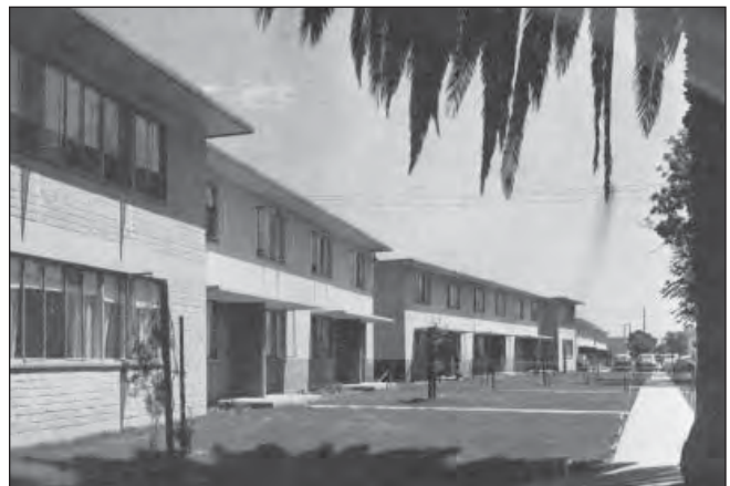
Low-slung buildings at Pueblo Del Rio, c. 1942 (from Homes for Heroes )
