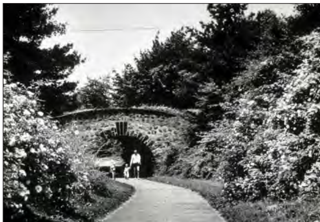
A pedestrian underpass at Radburn, which furthered the goal of keeping pedestrian and automobile traffic separate (Cornell University, Special Collections)
