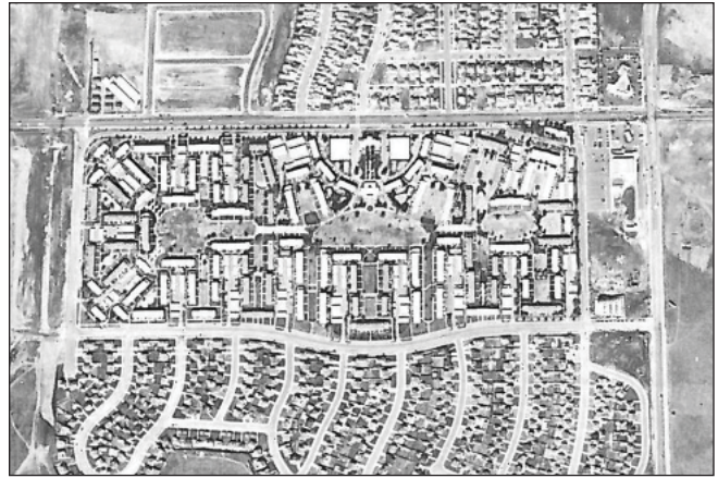
A c. 1948 aerial photograph of Baldwin Hills Village, showing its superblock site plan in contrast to the speculative development which grew around it (from Stein, Toward New Towns... )
