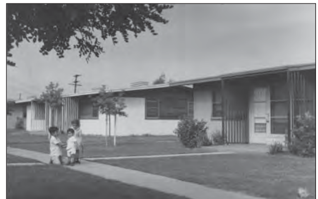
The landscape at Hacienda Village, shown here circa 1950, was designed by Ralph Cornell (Southern California Library for Social Studies and Research)
