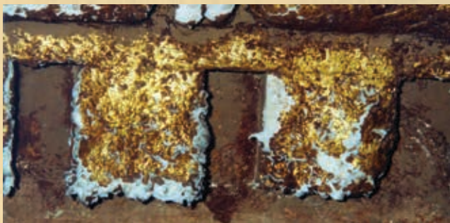
Prior to restoration, decorative plaster in the sanctuary was covered in a powdery efflorescence due to water and humidity damage. Photo courtesy of Simpson Gumpertz & Heger.
