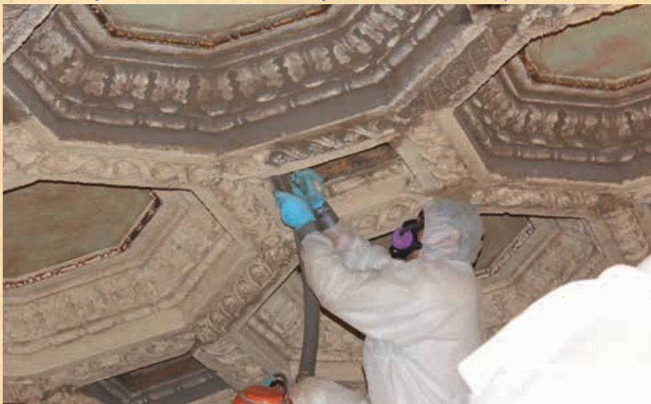
Each octagonal coffer on the dome was covered with over 80 years of built-up dirt and had to be carefully hand-vacuumed. Photo courtesy of Wilshire Boulevard Temple.
