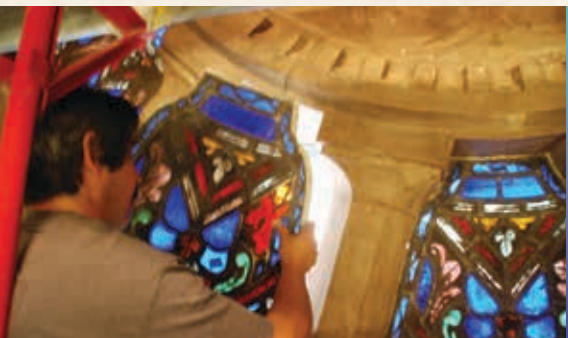
Above: The restored west tripartite window. Photo courtesy of Tom Bonner Photography. Below: Sections of the windows were carefully removed, inventoried, documented, cleaned, and repaired. Left photo courtesy of Judson Studios. Right photo courtesy of Levin & Associates Architects.
