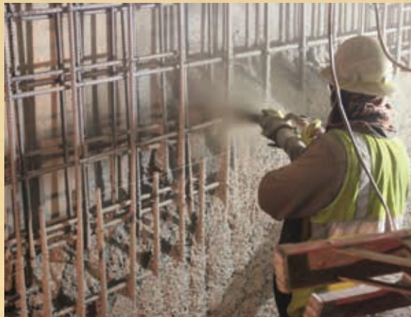
A member of the restoration team sprayed concrete through a hose at high velocity onto new shear walls as part of the seismic retrofit of the sanctuary. Photo courtesy of Wilshire Boulevard Temple.
