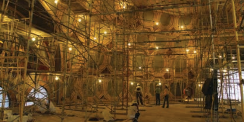
Scaffold platforms enabled the restoration team to work high above the sanctuary floor. Photo courtesy of Levin & Associates Architects.
