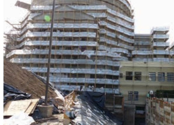
To repair exterior damage, scaffolding was erected all around the Temple and the parking lot was dug up to allow access to the basement to install the new HVAC system. Photo courtesy of Levin & Associates Architects.
