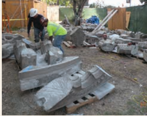
Members of the restoration team examined pieces of the stone casting that surrounded the Rose Window after it was removed for repair. Photo courtesy of Levin & Associates Architects.
