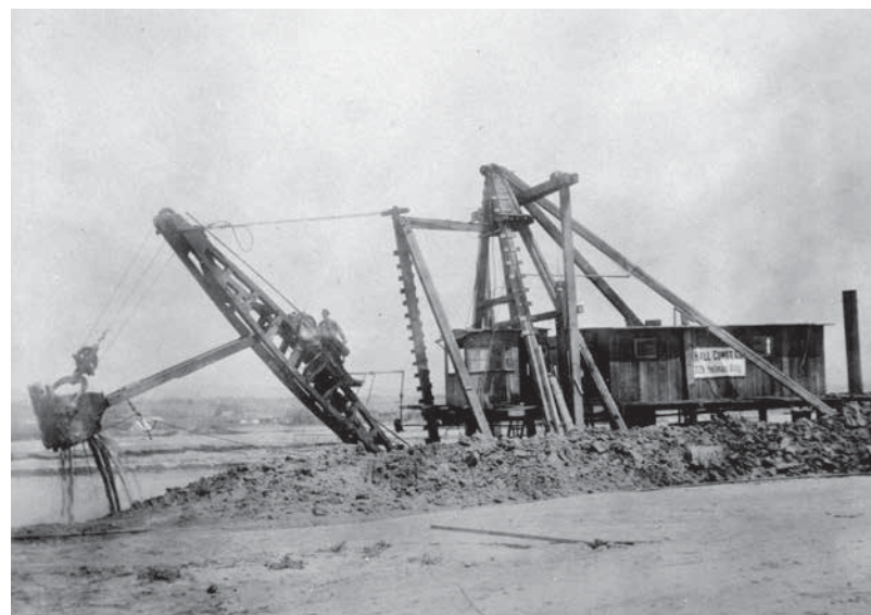
View of a dredger digging the Grand Canal in Venice, 1905.
