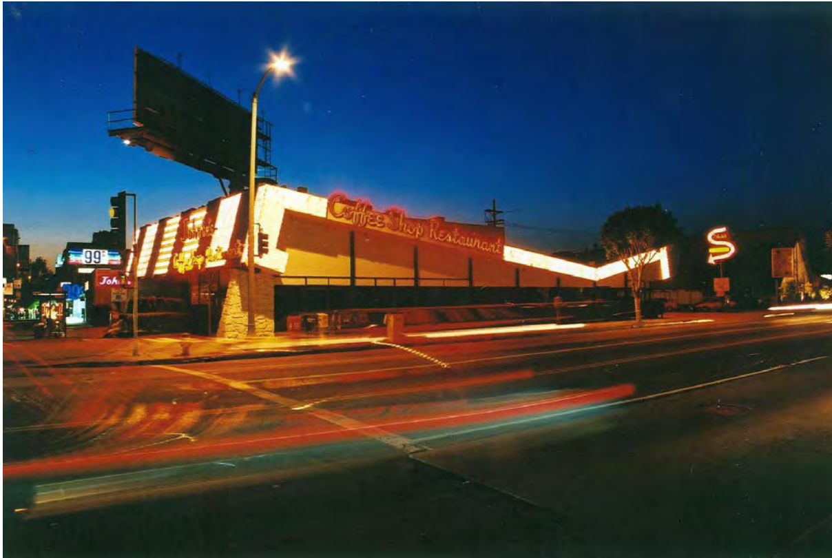
1. Johnie's Coffee Shop Restaurant, view looking northwest, front and east elevation. (Photo by John Eng, 2005)
