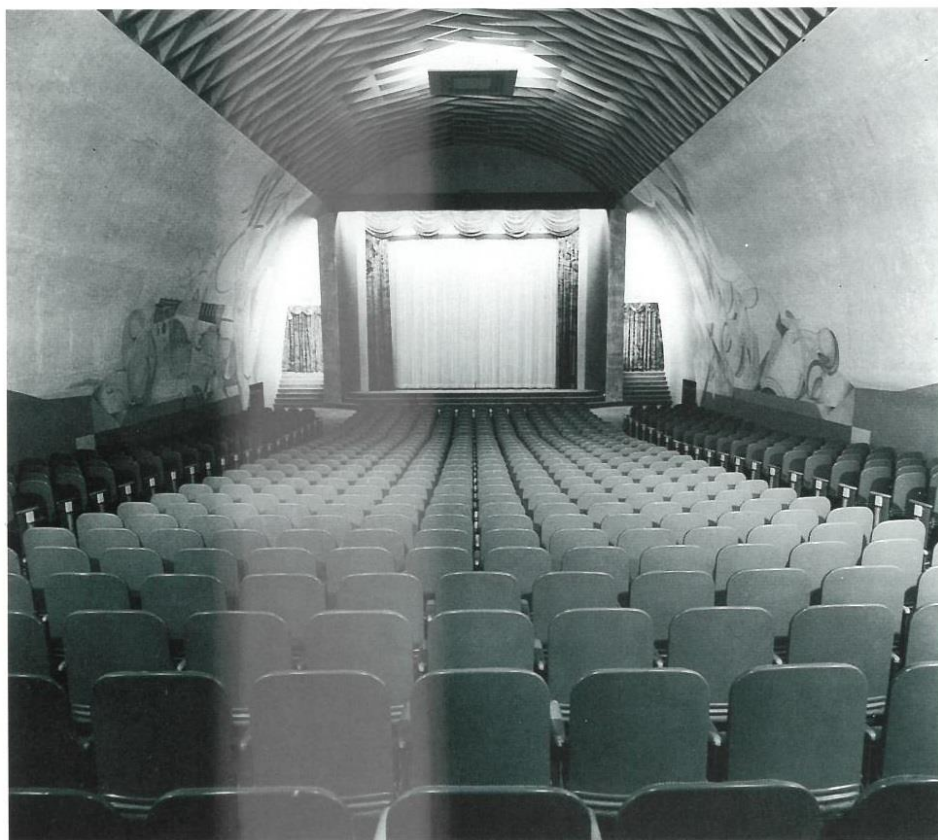
120 Puente Theatre, 1948. Auditorium with exposed lamella roof.
