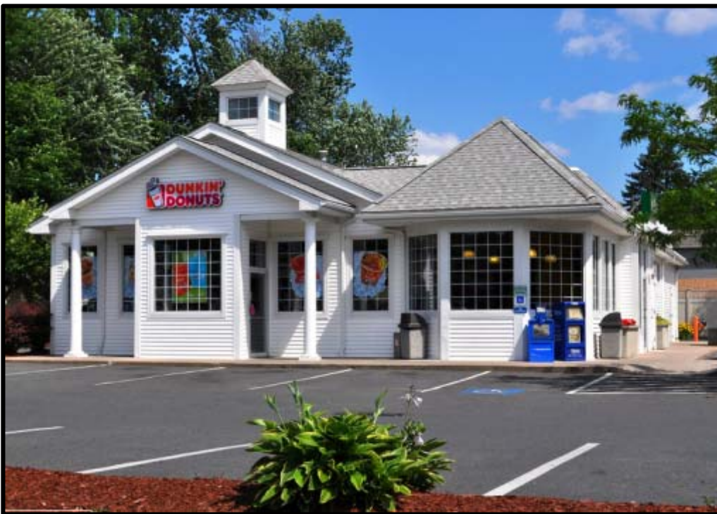
EXAMPLE: Dunkin' Donuts building designed to reflect local community character, North Elm Street, Westfield, MA.
