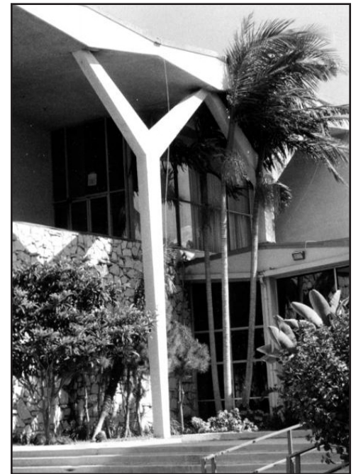
The "Y" shaped piers of the main building are one of the hotel's distinctive elements.
