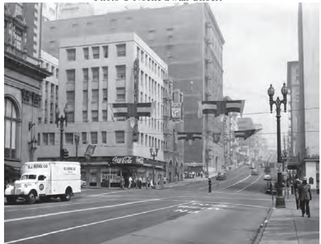
San Carlos Hotel on the left (Coca Cola). Initially the Auditorium Hotel 1904-1929 - Renamed San Carlos Jan 1929 - Demolished 1987 View up Olive St near 5th St. Biltmore near left. John R. Leff, Security Pacific National Bank Collection, Los Angeles Public Library photos.lapl.org
