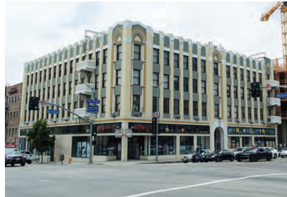
Current View of Mayer Building Photo: Noelle Swan Gilbert
