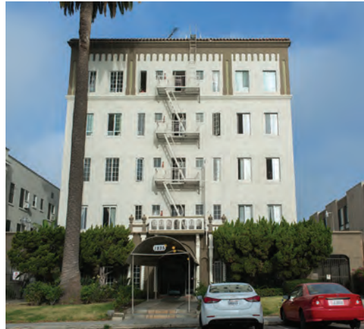
Present Day View of Neff Apt Building Photo©Noelle Swan Gilbert
