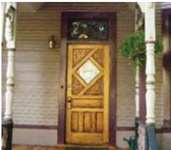
The narrow door with a transom window above is common in Victorian architecture.
