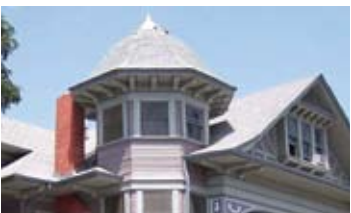
The varying roof forms, including a turret (round tower), set this home apart.
