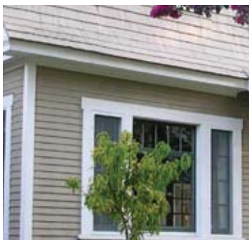
Some buildings like this one have two types of siding, lap siding on the bottom and shingles on top.
