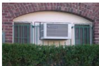
The original arched opening has been filled in with an air conditioner and smaller windows.
