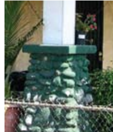
The river rock on the base of the columns should not be painted.
