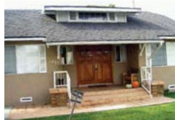
This door opening has been altered to install double doors.
