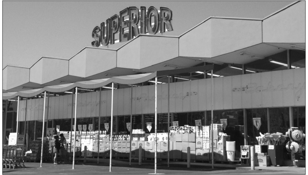
The owner of this supermarket plans to destroy the Googie façade and give it a Craftsman-like makeover. Photo by Cindy Olnick/L.A. Conservancy.
