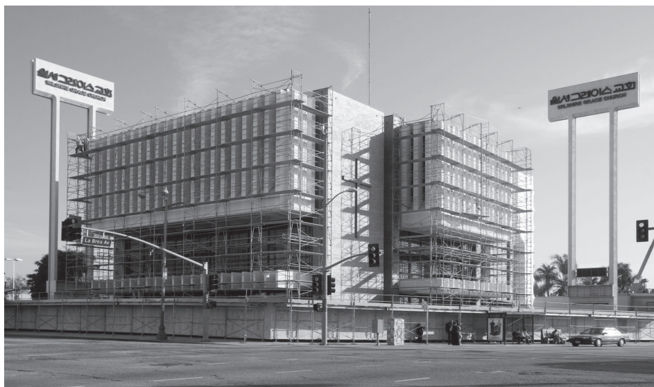
Scaffolding goes up around the Columbia Savings Building in preparation for its demolition. Photo by Larry Underhill.
