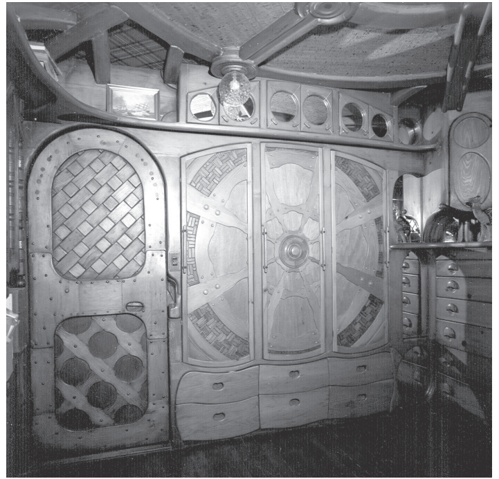
The Conservancy holds an easement protecting the original landscaping, exterior façade, and interior features (pictured) of the Joseph Residence and Apartments (1946-70). Photo by Larry Underhill.
