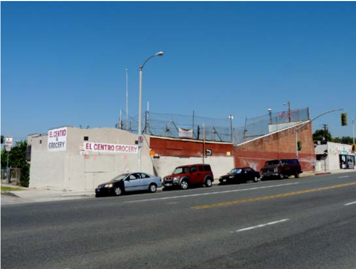
View of east façade of Maravilla Handball Court and El Centro Grocery.
