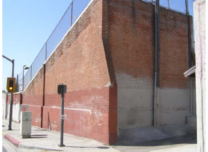
View of original north and east walls of Maravilla Handball Court.
