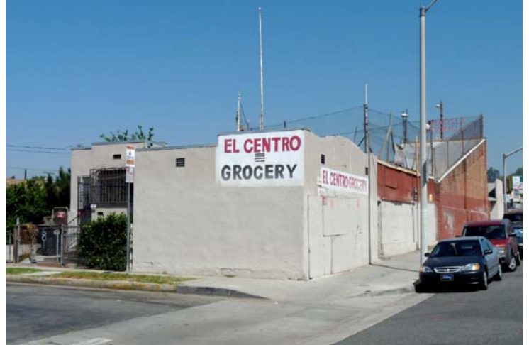
South façade of El Centro Grocery.
