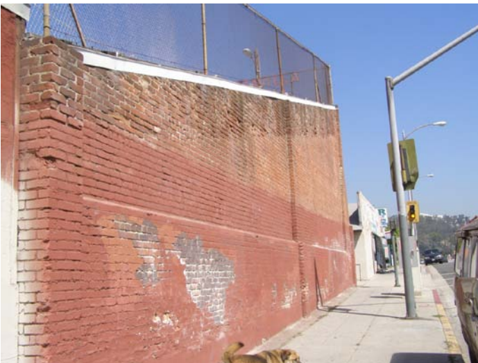
East façade of handball court, view looking north.
