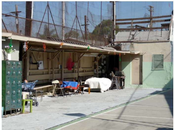
Interior of west wall and storage building at northwest corner of handball court.
