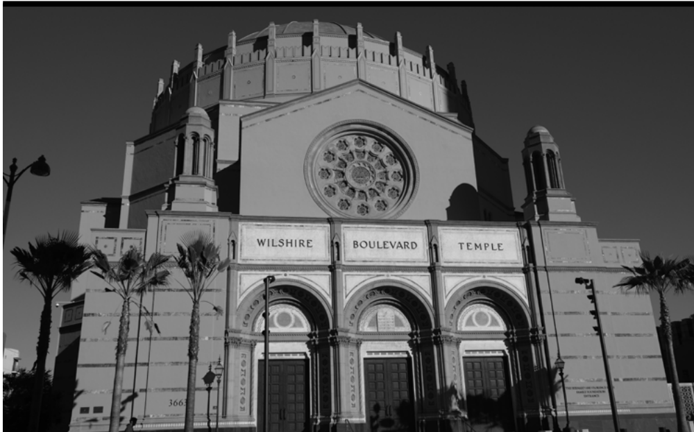
The Conservancy's tour of Wilshire Boulevard Temple will take place on Sunday, April 27. Photo by Adrian Scott Fine/L.A. Conservancy.
