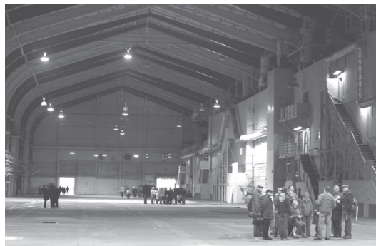
Guests visit Building 15, one of the largest wooden structures in the world. Photo by Greg Szimonisz.
