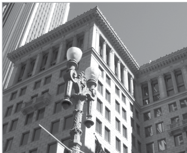
PacMutual recently became the oldest building in Southern California to earn LEED Platinum certification. Photo by Annie Laskey/L.A. Conservancy.
