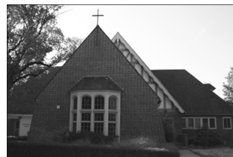
This chapel on the Fred C. Nelles Youth Correctional Facility campus was built between 1930-1933. Photo courtesy Whittier Conservancy.
