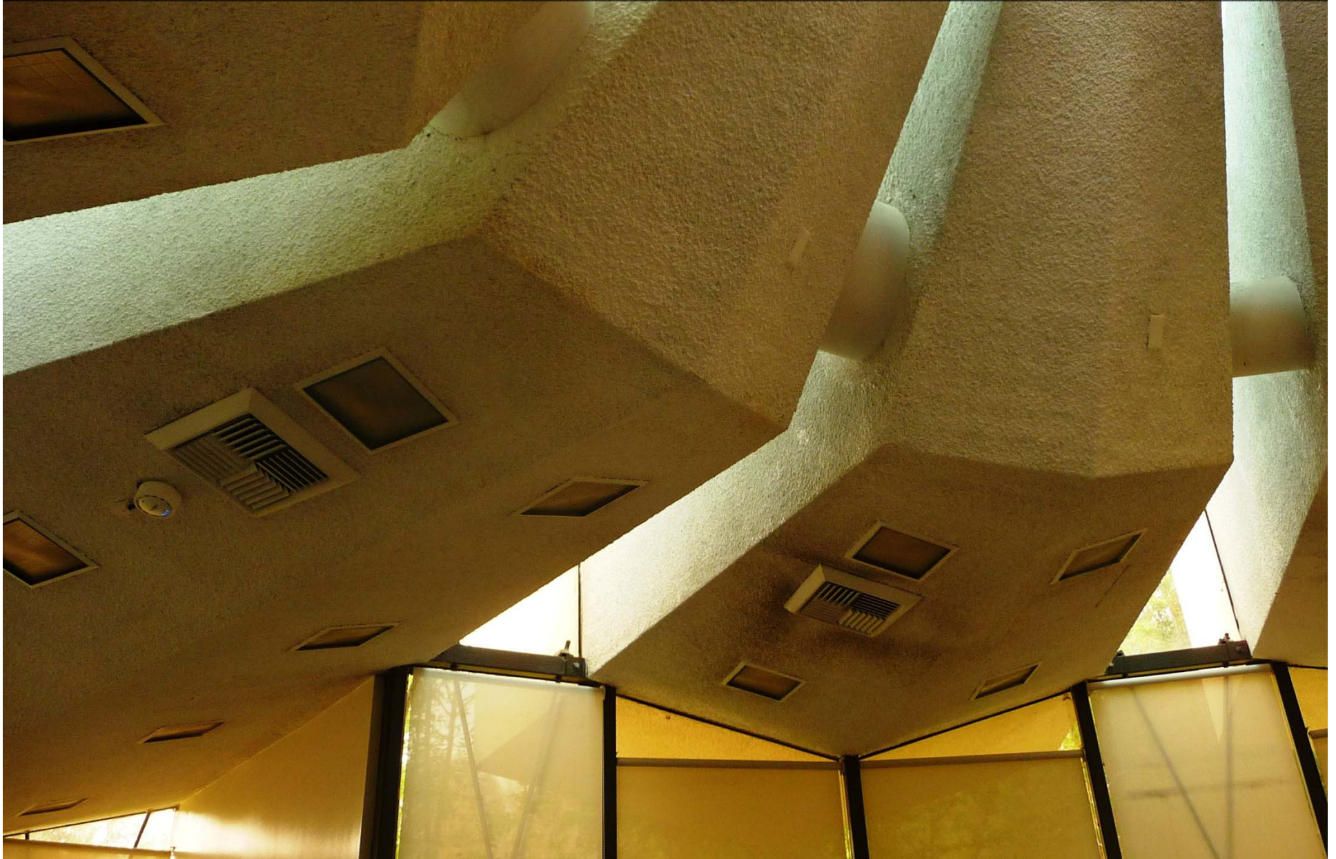
John Lautner-designed Crippled Children's Society Rehabilitation Center (in 2013) 6350-60 Winnetka Avenue Courtesy: Los Angeles Conservancy / Submitted May 20, 2014
