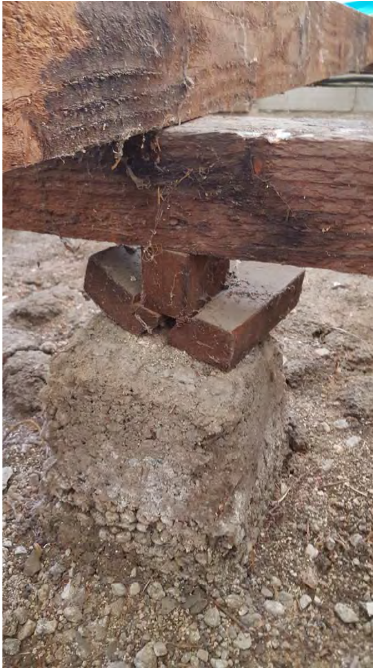
Failed Foundation Shim and Poor Concrete Quality of Pier
