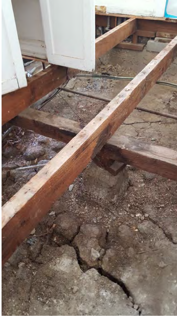
Floor Framing in Northwest Unit Exposed with Cracked Shallow Fill Soil
