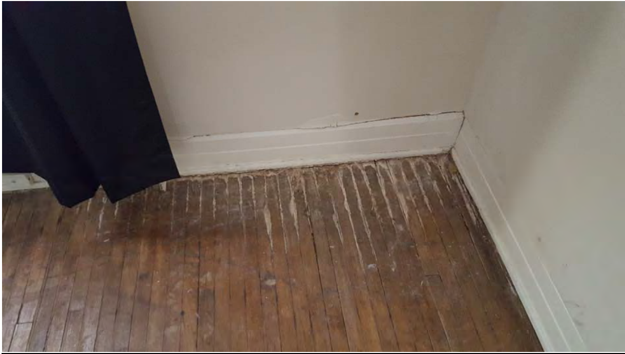
Interior Water Damage and Settlement
