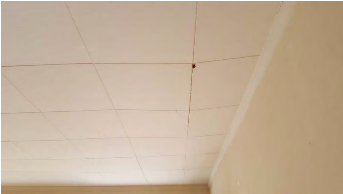
Interior Ceiling Damage from Settlement
