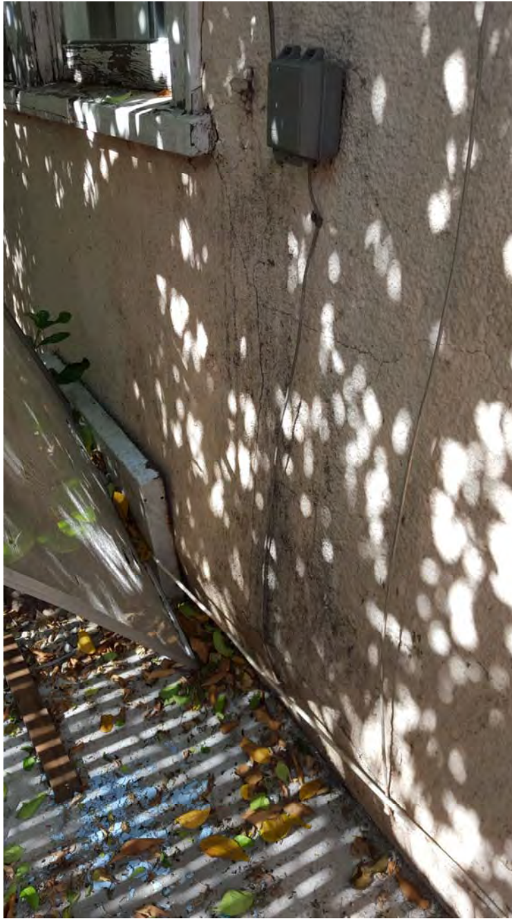
Significantly Bulging Cripple Wall
