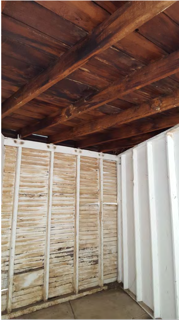
Damaged Garage Roof Framing and Wall Straight Sheathing
