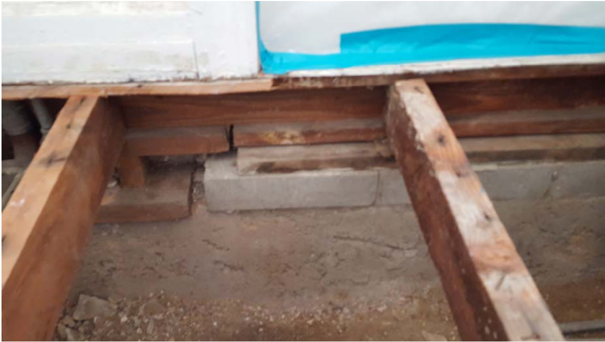
Hybrid Wood/Masonry Sill Plates Missing Bolting
