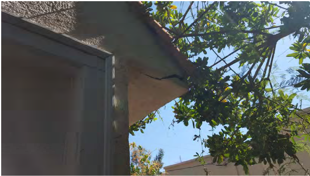
Damaged Eave
