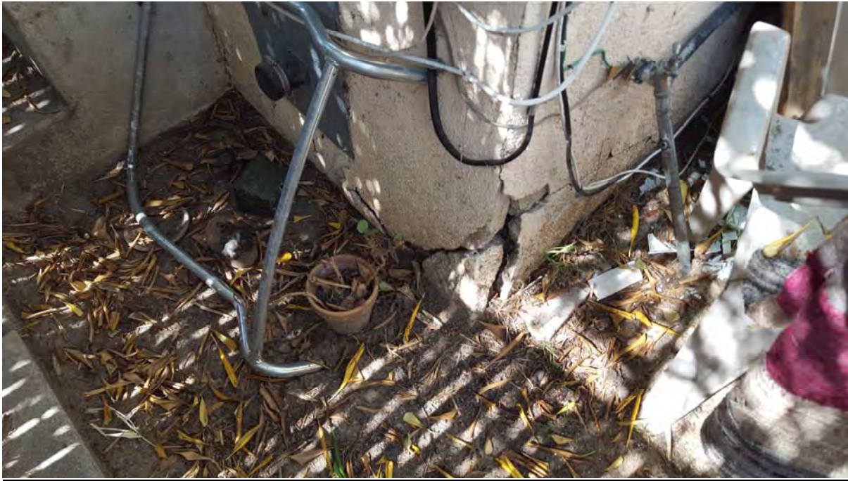
Failed Stucco at Corner
