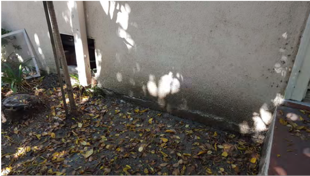
Bulging and cracked foundation stem wall
