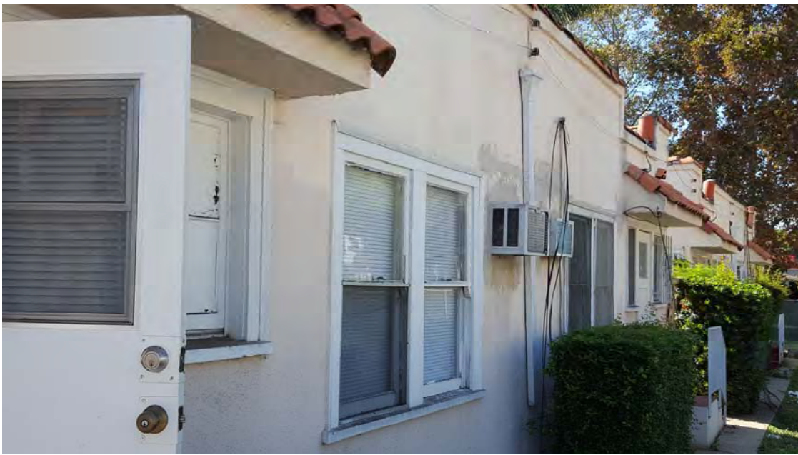
Added Opening in Stucco Wall reducing Seismic Capacity
