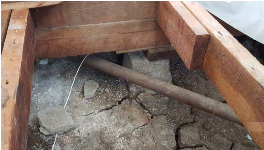
Heaved and Settled Foundation Pier
