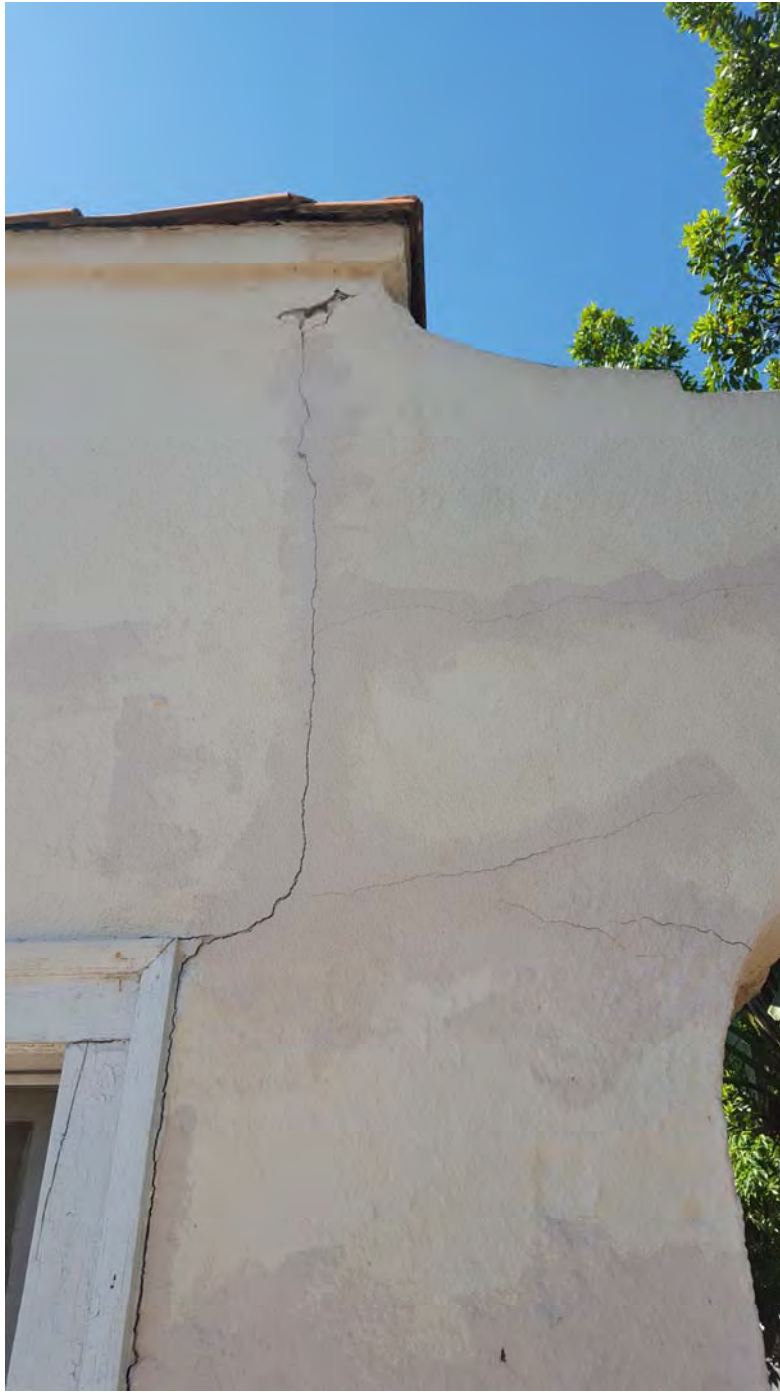
Typical Exterior Plaster Cracks
