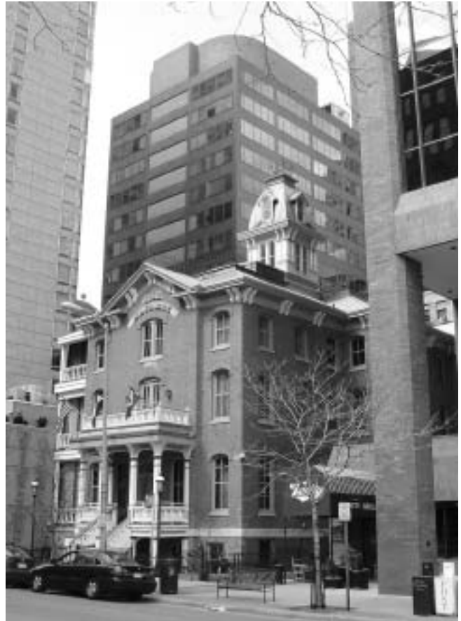
Several buildings in Denver, Colo., have taken advantage of the city's TDR program including the Navarre Building (pictured here), the Denver Athletic Club, and the Odd Fellows Hall.
