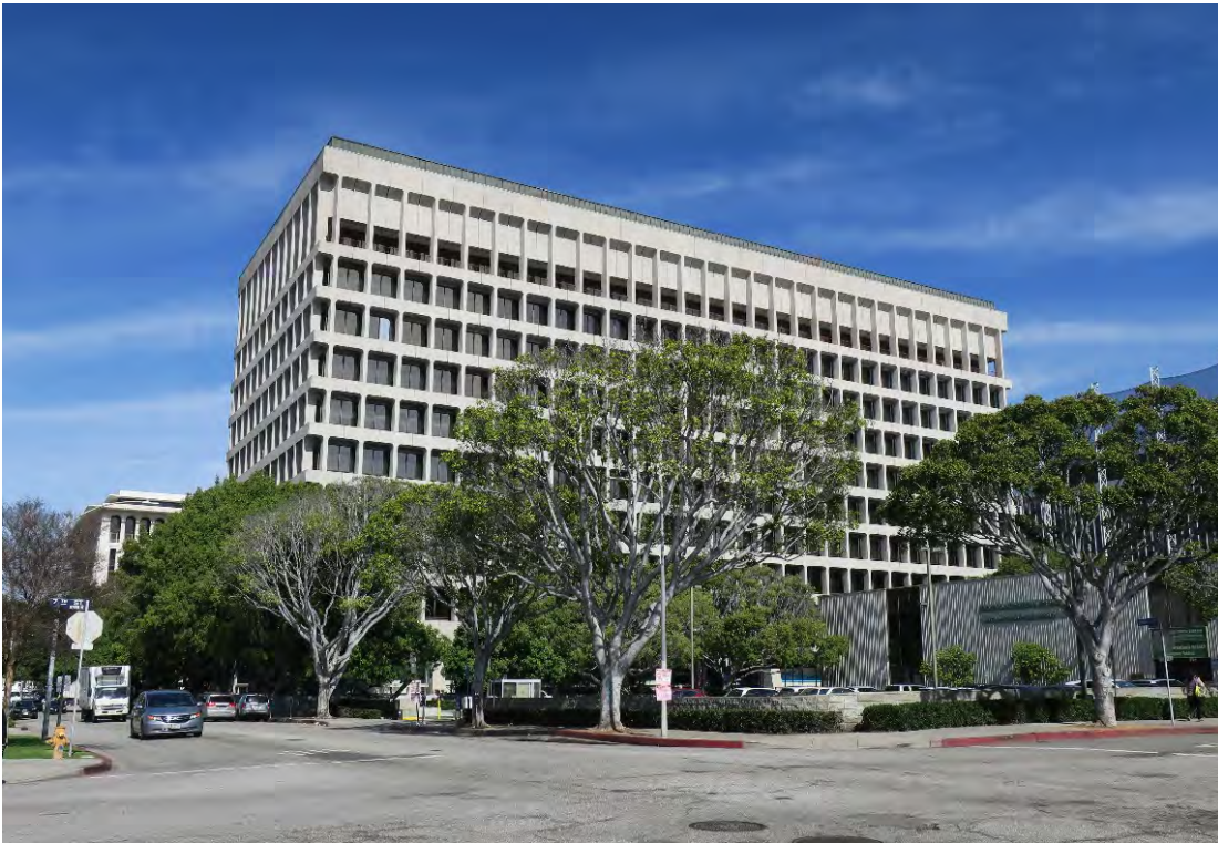
South façade and setting, view northeast (ARG, 2017).
