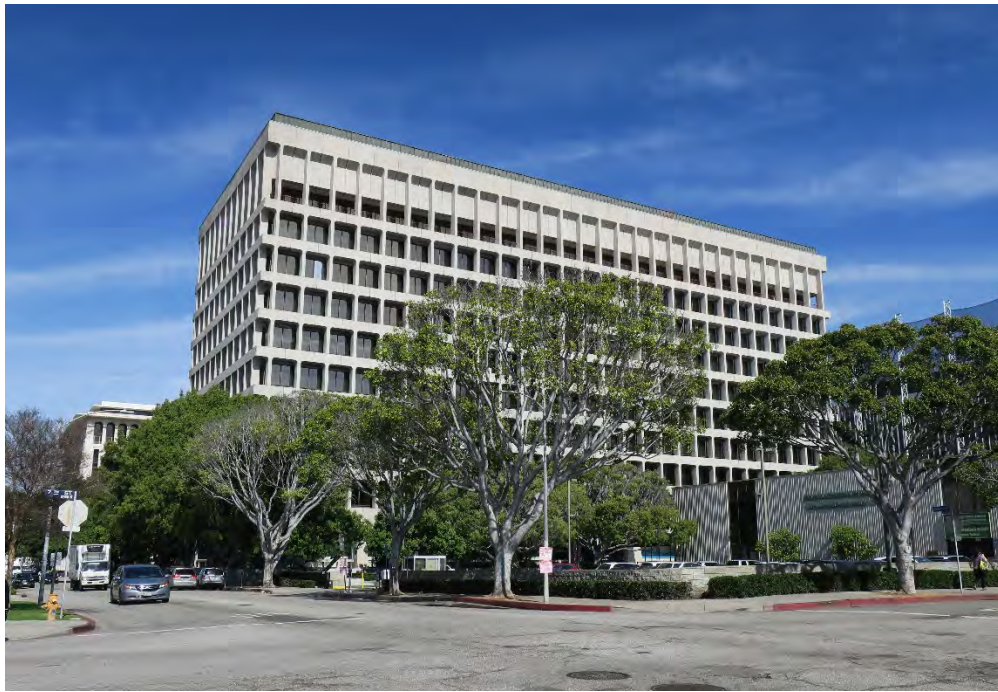
South façade and setting, view northeast (ARG, 2017).
