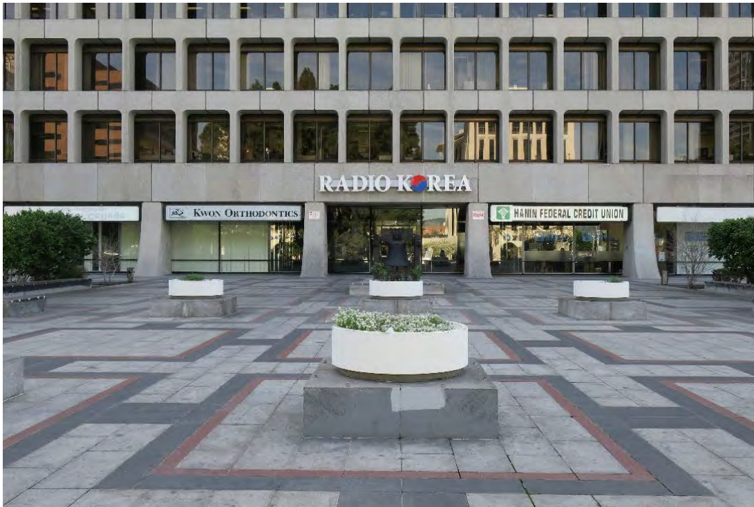
Bottom portion of north façade and hardscaped plaza, view south (ARG, 2017).
