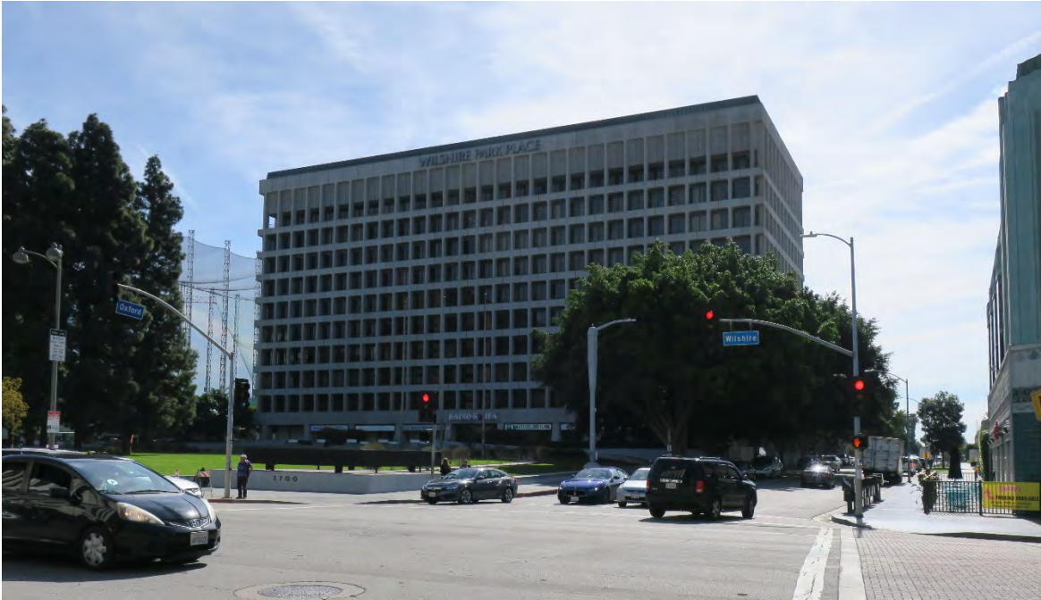
Primary (north) façade and setting, view southeast (ARG, 2017).
