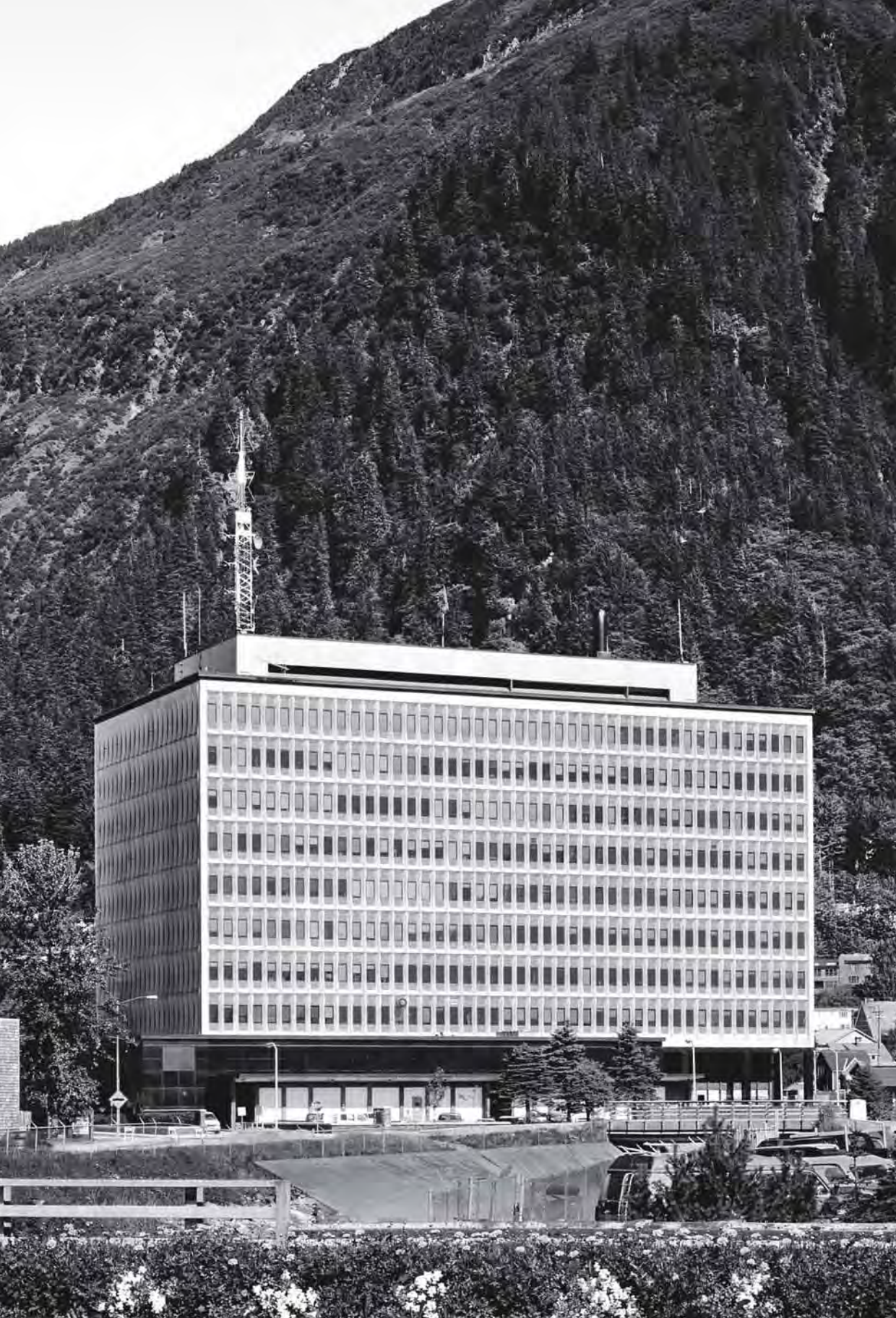
HURFF A. SAUNDERS FEDERAL BUILDING. U.S. POST OFFICE AND COURTHOUSE. JUNEAU, ALASKA | OLSEN & SANDS | 1966
