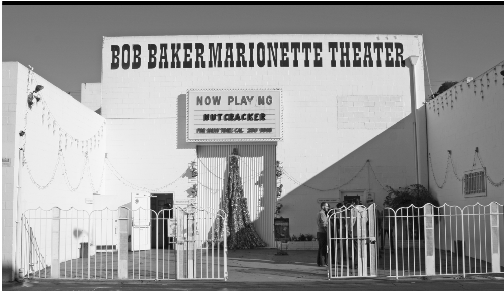
While this modest building is unspectacular architecturally, it is culturally significant for the key role it played in the history of puppetry. Photo by Jessica Hodgdon/L.A. Conservancy.
