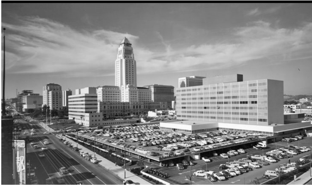
The City of Los Angeles, through its Bureau of Engineering, is seeking to demolish Parker Center and replace it with one or two high-rise towers. The Conservancy believes that this historic building can be incorporated into a new construction project, preserving its history and saving millions of taxpayer dollars. Undated photo of Parker Center and Los Angeles City Hall, courtesy of Security Pacific National Bank Collection/Los Angeles Public Library.
