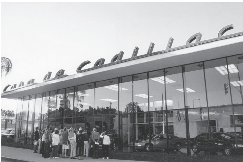
Casa de Cadillac (1949), Sherman Oaks. Photo by Larry Underhill.
