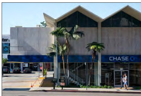
Lytton Savings' dramatic, folded-plate concrete roof was a striking departure from traditional bank design when it was constructed in 1960. Photo by Hunter Kerhart.
