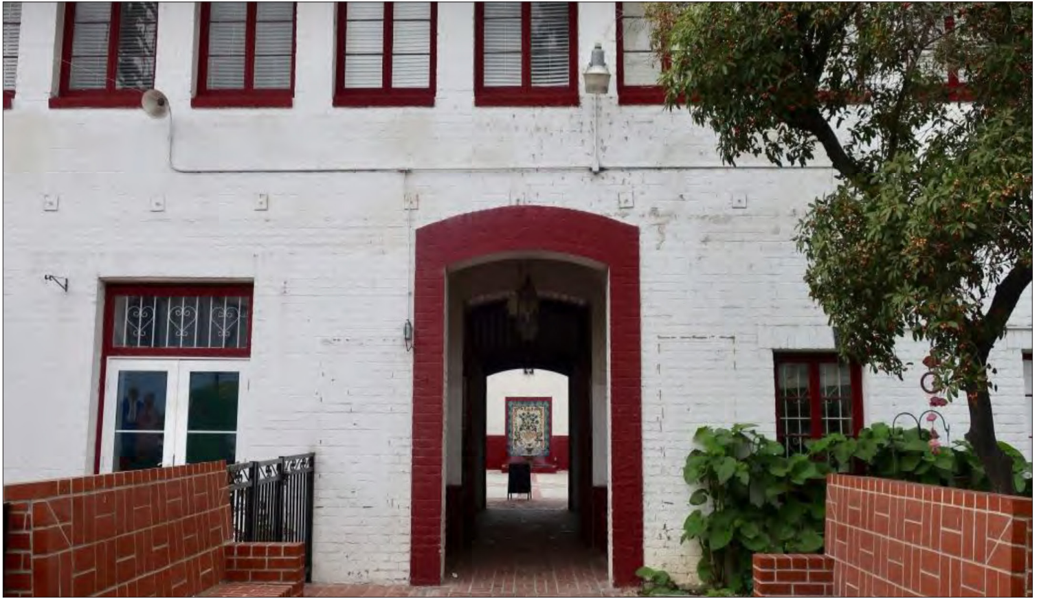
Exterior of the International Institute's administration building in Boyle Heights, 2017. This Spanish Colonial Revival style building debuted in 1932. Photo by Laura Dominguez
