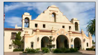
San Gabriel Mission Playhouse, one of many historic resources in San Gabriel. Photo courtesy SWCA Environmental Consultants.
