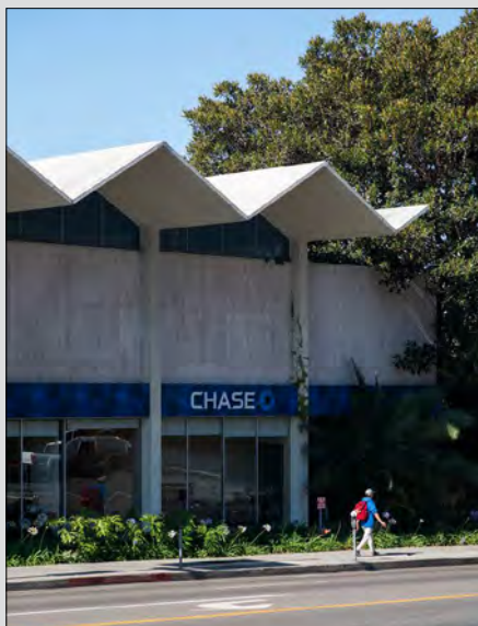
This Modern bank building's folded-plate concrete roof is one of its most distinctive features. Photo by Hunter Kerhart.
