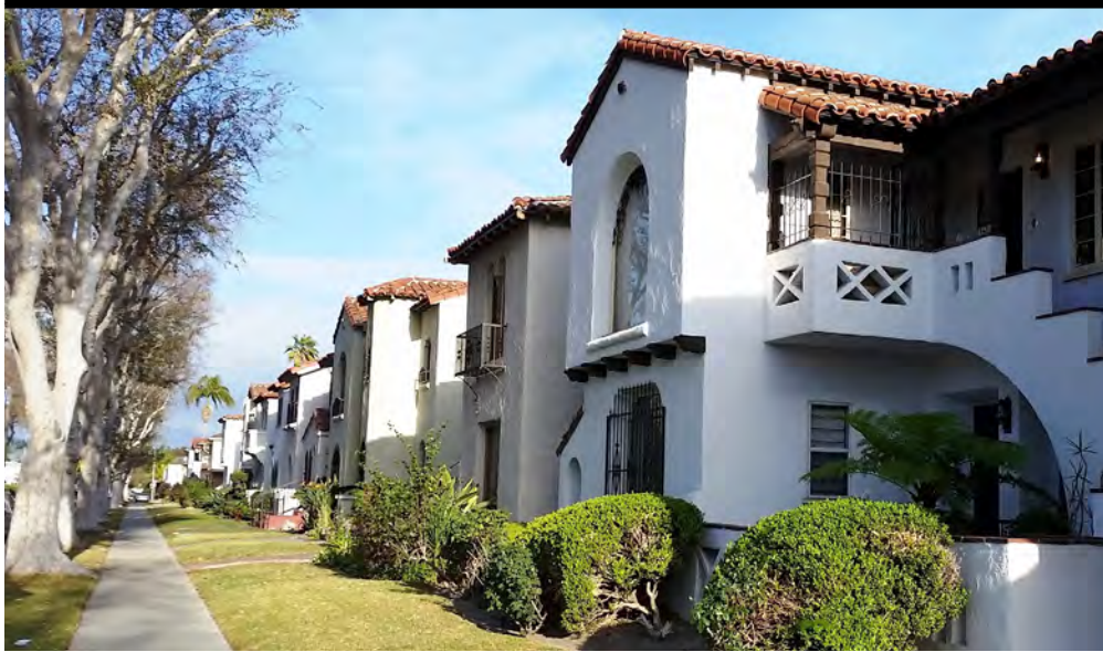
In June of this year, the City of Los Angeles adopted a new West Adams-Baldwin Hills-Leimert Park Community Plan. The plan identifies the historic Leimert Park neighborhood as an area warranting preservation and neighborhood conservation strategies. Photo by Adrian Scott Fine/L.A. Conservancy.
