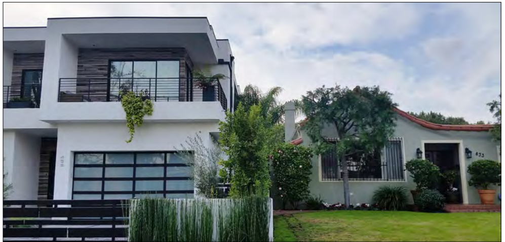
More than any other design element, bulky, front-loaded, attached garages severely alter the overall character of an older neighborhood. A loophole in the Baseline Mansionization Ordinance has led to many incompatible designs appearing in older and historic neighborhoods. Photo by Adrian Scott Fine/L.A. Conservancy.
