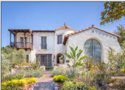
One of the homes we will visit on the tour is the 1928 Spanish Colonial Revival-style James Doumakes Residence. This private home was the first house in unincorporated L.A. County to gain landmark status. Photo courtesy deasy/penner&partners.
