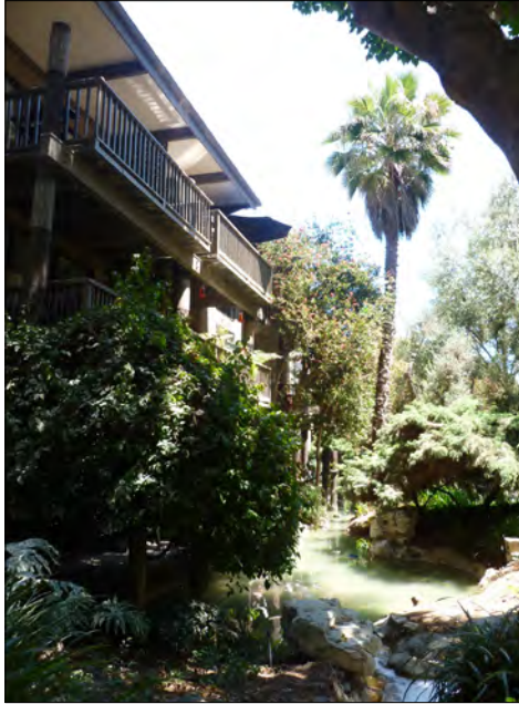
A proposed renovation project would remove original plantings and water features at the Mariners Village apartment community in Marina del Rey. Photo by Katie Horak.
