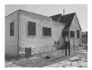
This rear view of one unit illustrates the tiled parapet roof and clay pipe vent holes, as well as the steeply pitched Tudor style roof.
