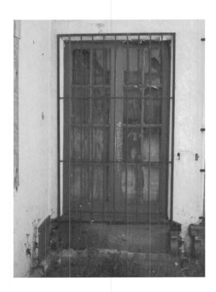
Some units have French doors that open into the "court." The decorative wood scrollwork below the threshold is severely deteriorated and non-existant on some units.
