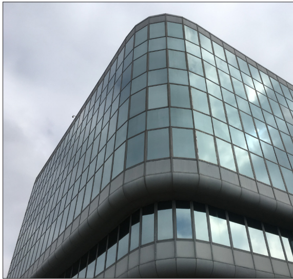
The FAA building features a rounded, taut glass-and-aluminum-skinned façade. Photo by Adrian Scott Fine/L.A. Conservancy.
