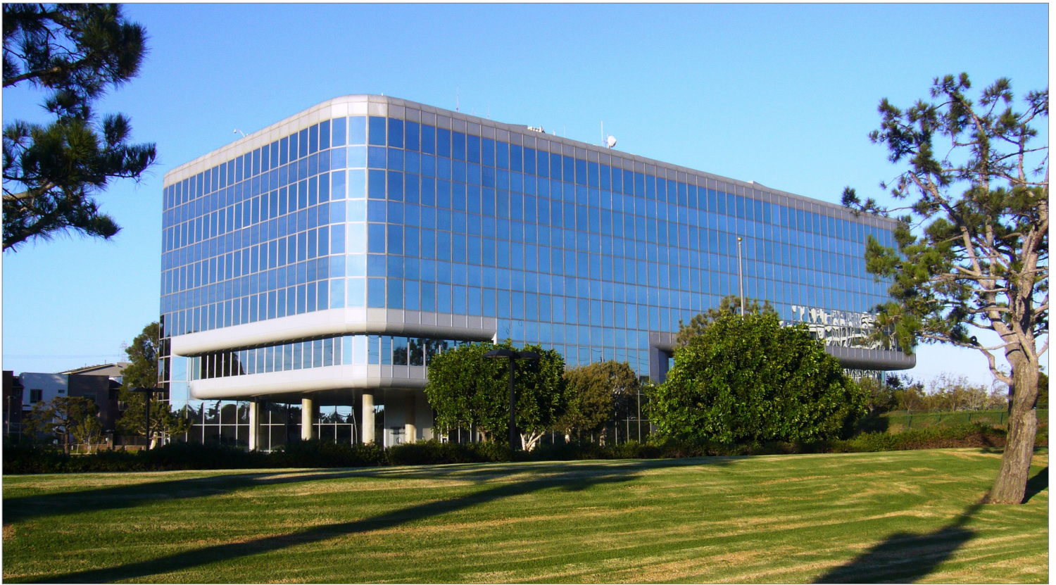
The 1972 Federal Aviation Administration Building (FAA) in Hawthorne is protected by an easement held by the Conservancy. Photo by Adrian Scott Fine/L.A. Conservancy.
