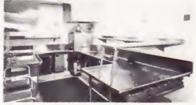
Showing stainless steel kitchen equipment planned by Norman Roybark. The V-shaped glass wall and stainless steel equipment would permit cleaning this kitchen with a steam fire, very little smoking in dining room and this results primarily of cooking range. Steamings from food are disposed of in a bi-weekly disposer and table scraps are eliminated in separate disposal units.
