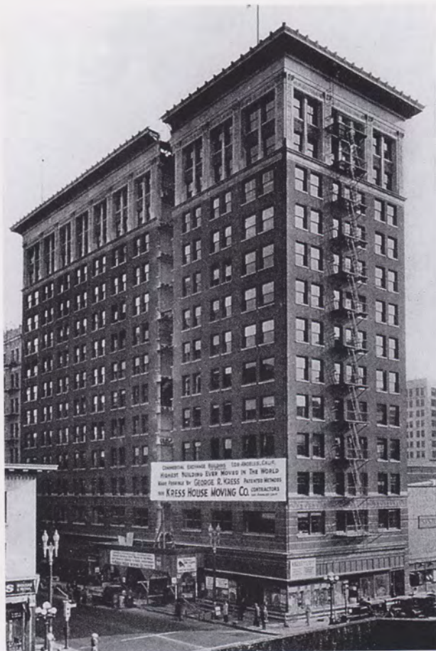
The 14-story Commercial Exchange Building was cut into two sections, a five-foot section removed, and the two remaining sections joined back together. It was considered one of the greatest engineering feats of its time. The George R. Kress Collection
