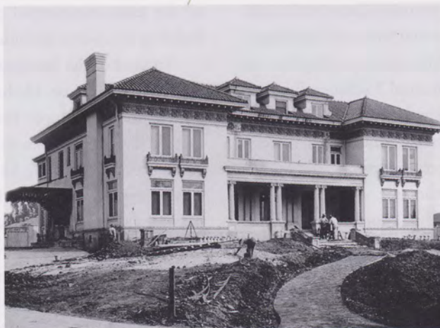
The Aaronson residence was moved from Wilshire Boulevard to Fremont Square. This two and one-half story, 40-room Beaux Arts-styled mansion was cut into three sections, each weighing 400 tons.
