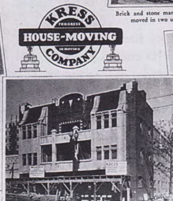
Three-story brick apartment building, 50x110, moved by the George R. Kress method.
