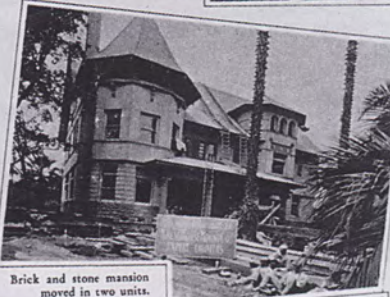
Brick and stone mansion moved in two units.
