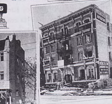
Section of four-story brick building moved with George R. Kress patent bracing devices.
