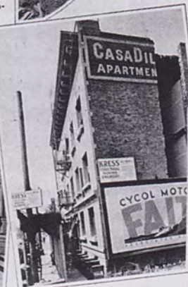
Section of building moved with same patent devices.
