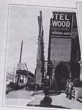
End view of wall moved by George R. Kress Patent devices.
