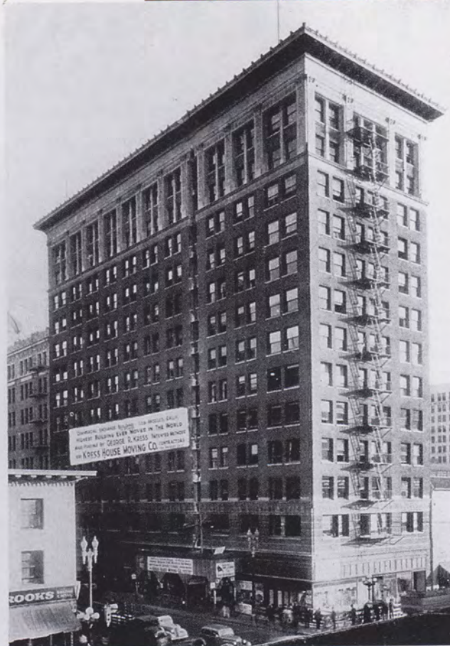
The 14-story Commercial Exchange Building was cut into two sections, a five-foot section removed, and the two remaining sections joined back together. It was considered one of the greatest engineering feats of its time. The George R. Kress Collection
