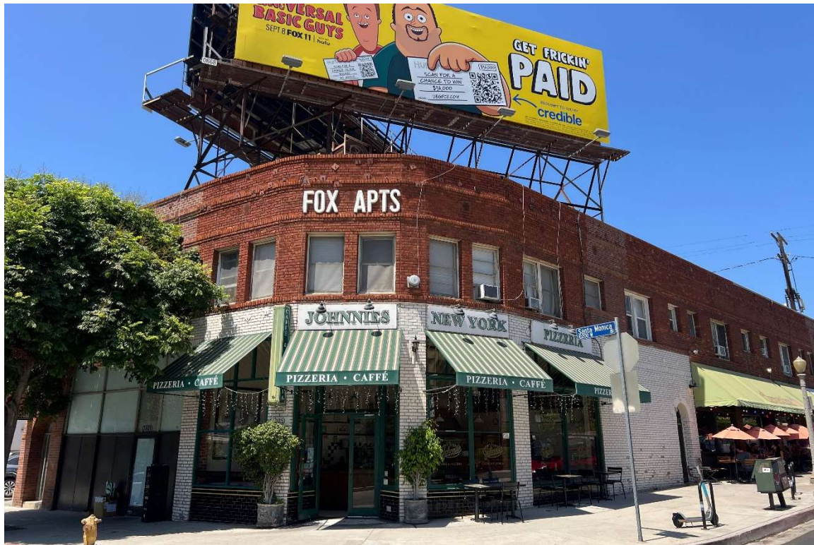
Photo 1: South and east façades, view northwest from Santa Monica Boulevard
