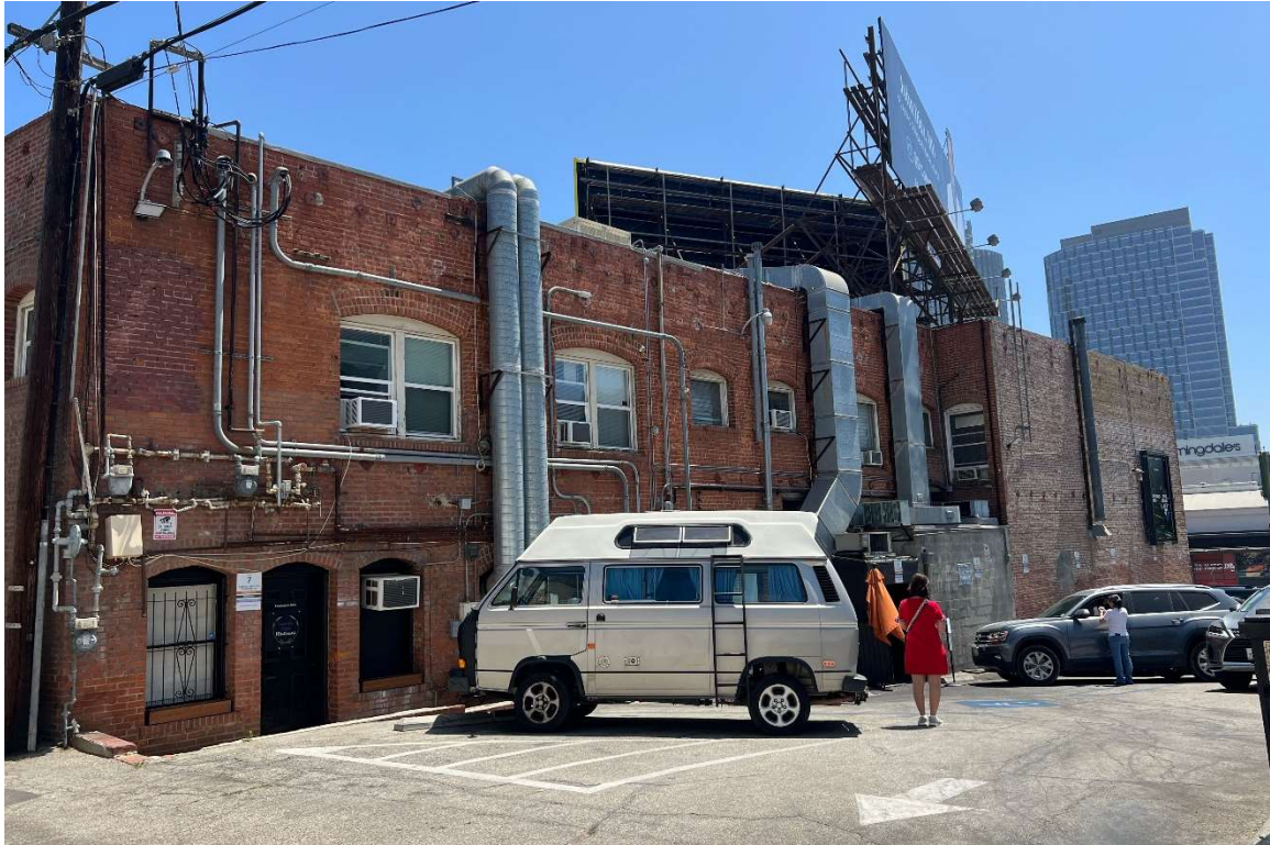
Photo 10: West façade, view southeast from alley
