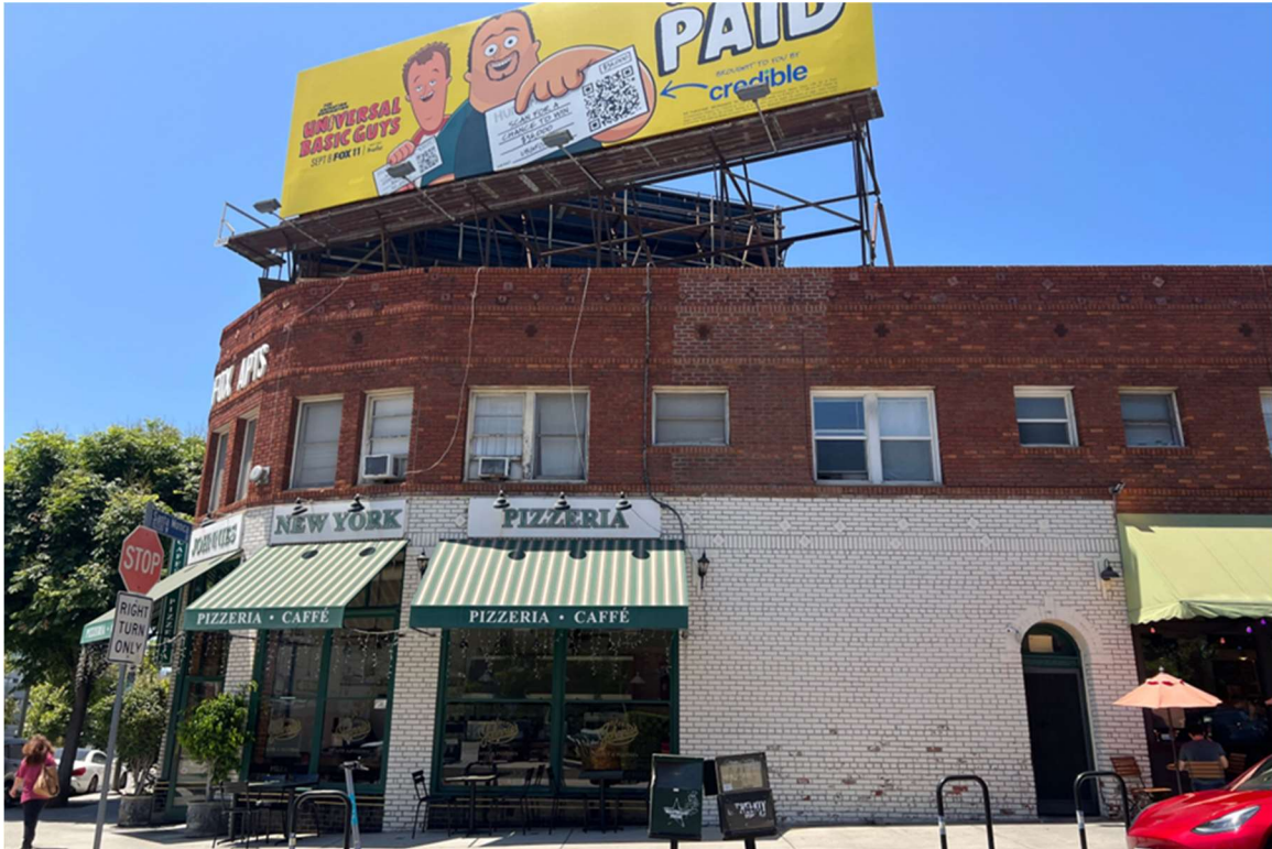
Photo 4: East façade, view west from Ensley Avenue
