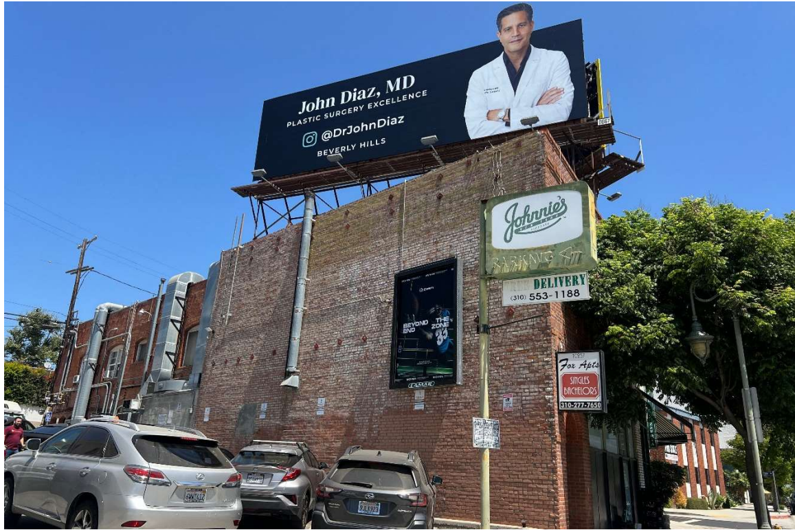
Photo 11: West façade, view northeast from Santa Monica Boulevard
