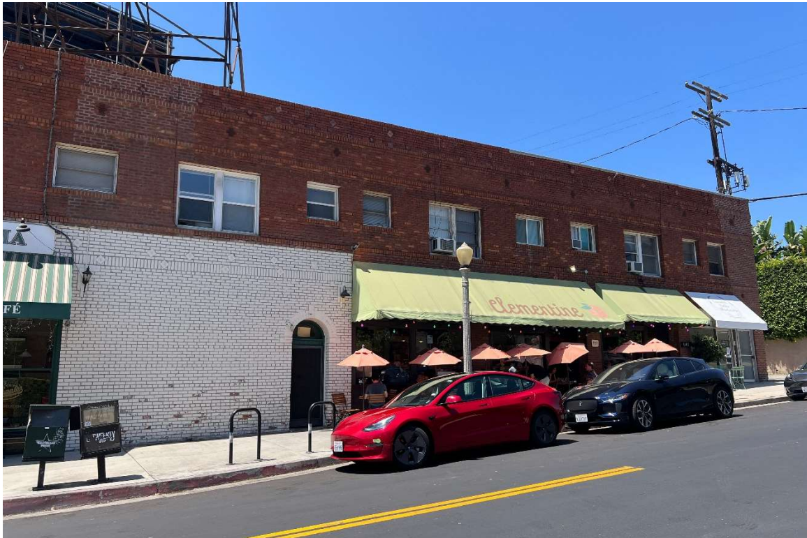
Photo 6: East façade, view northwest from Ensley Avenue
