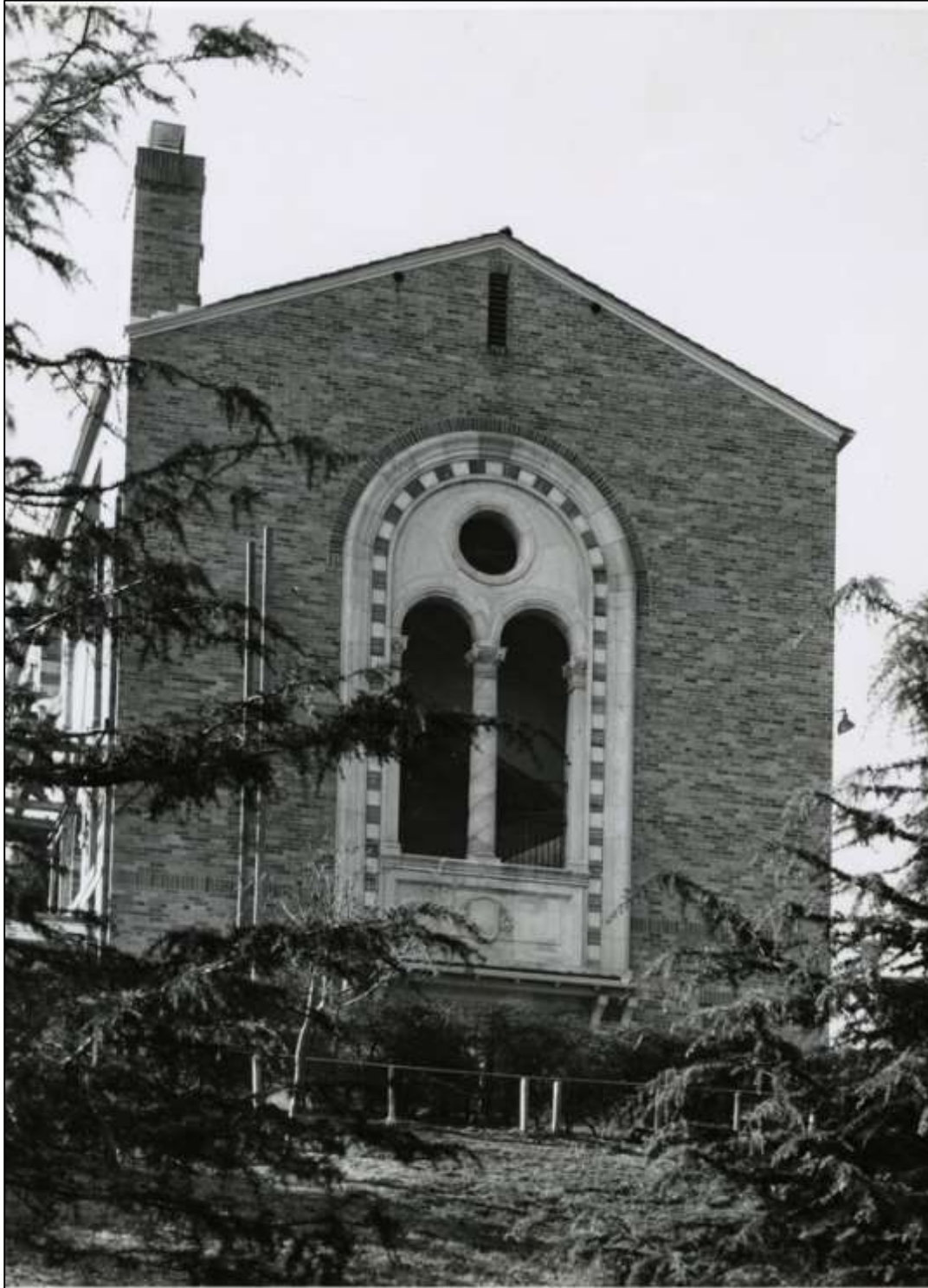
Figure 8 Venetian window after repairs following 1933 Long Beach Earthquake, circa 1936
